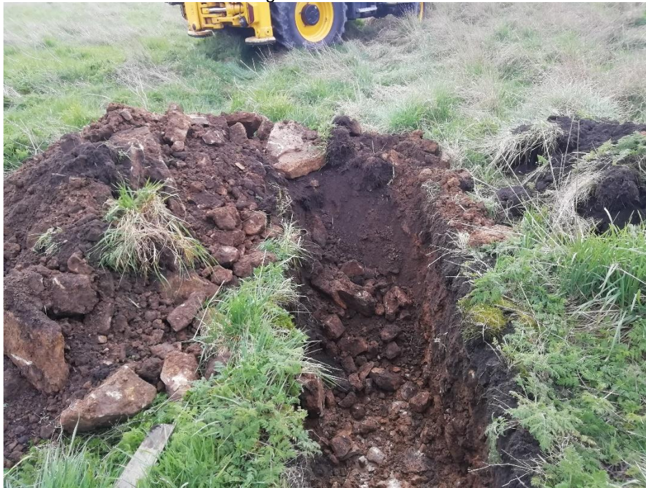
Figure 8: Trial Pit 3 Spoil
