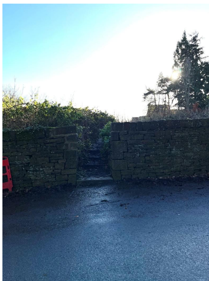
Photo 3.5: Pedestrian Access from Parkwood Road
