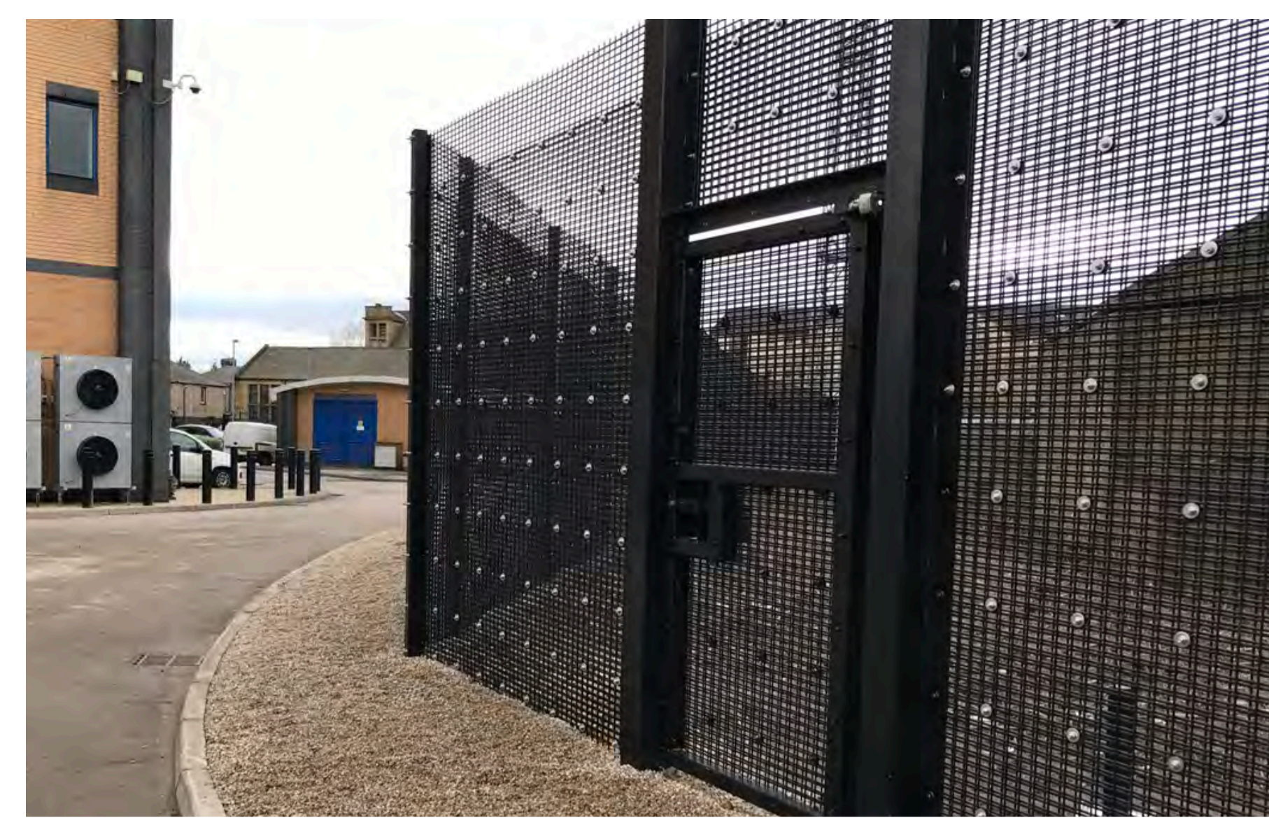
G1- 1.2m wide single leaf Pedestrian Gates UHS Extreme Mesh SR3 Height Overall to line through with fence to maintain perimeter security - over panel may be required
