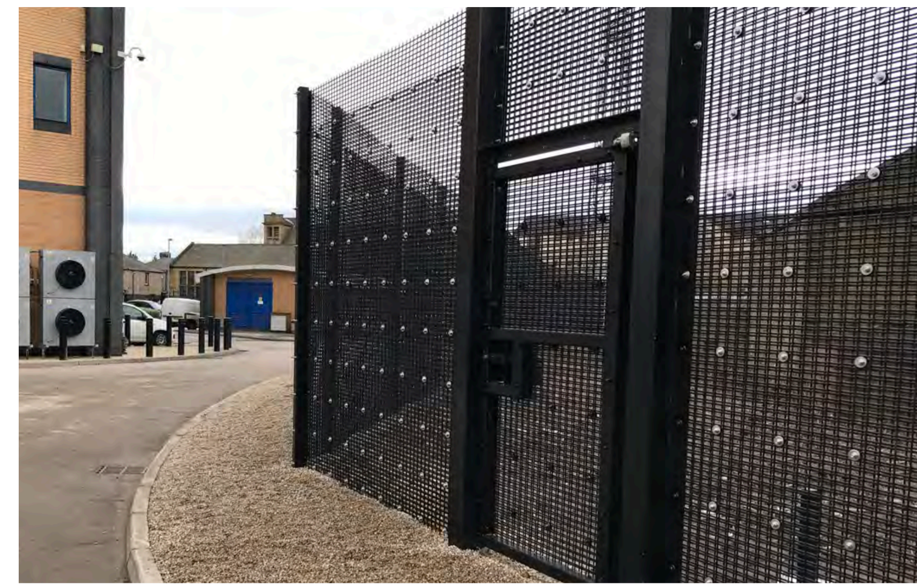
G1 - Pedestrian Gates UHS Extreme Mesh SR3 Height Overall to line through with fence to maintain perimeter security - over panel may be required
