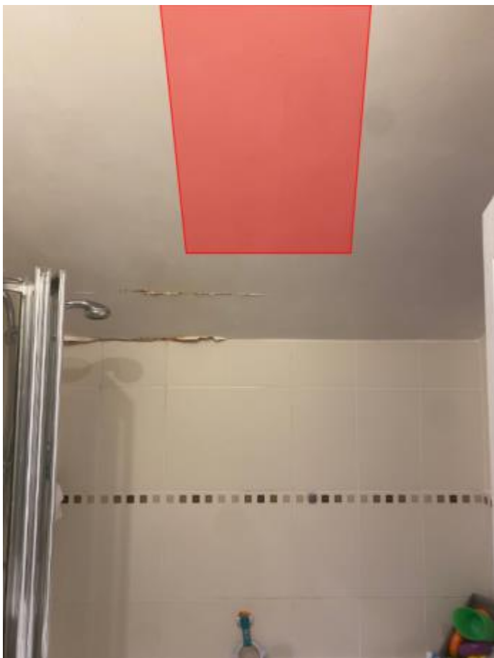
Approximate location of rooflight installation shown in red
