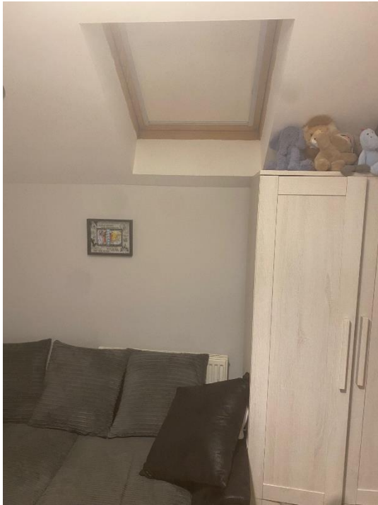
Existing rooflight in adjacent bedroom
