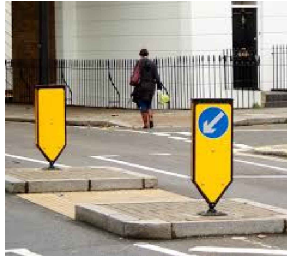
* PASSIVELY SAFE BOLLARDS
