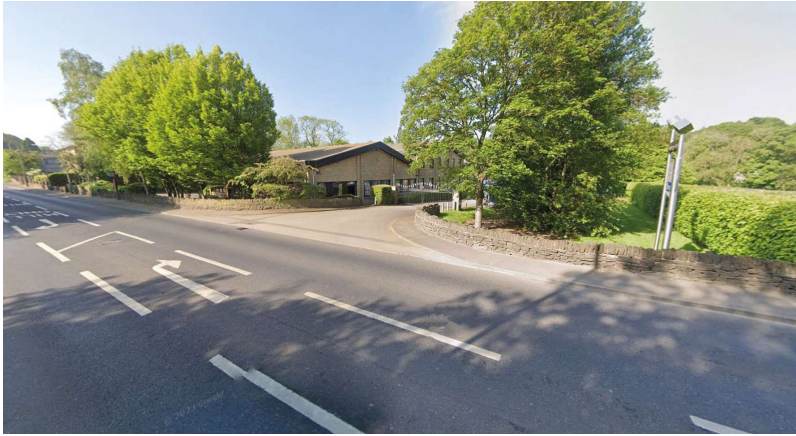
View One - View towards International House from Penistone Road
