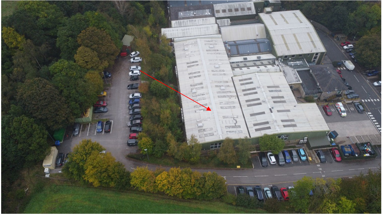
Building 1 is fully sealed
