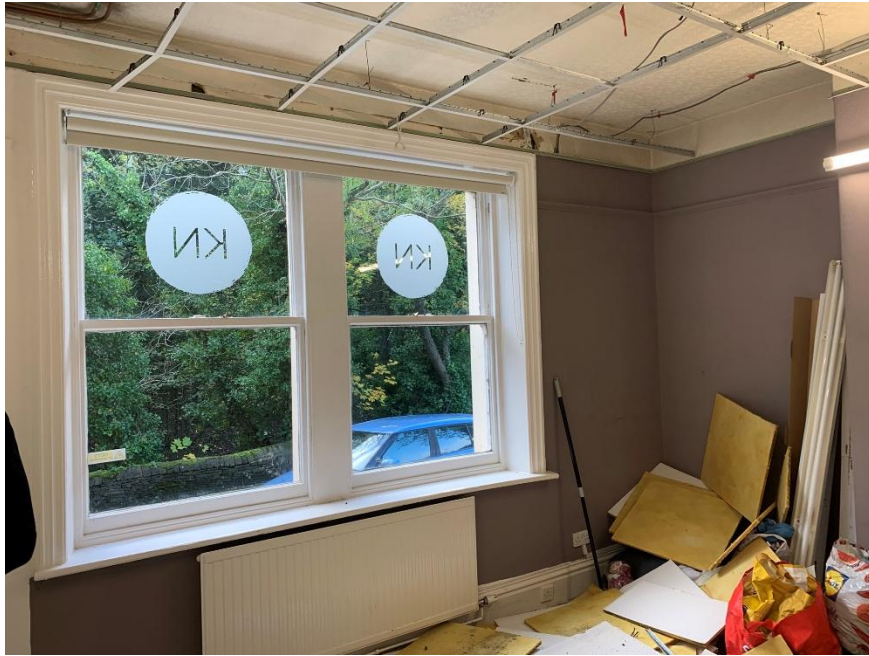
Photo 03 – Internal view, with suspended ceiling and window manifestation where the building was a Beauty Salon.
