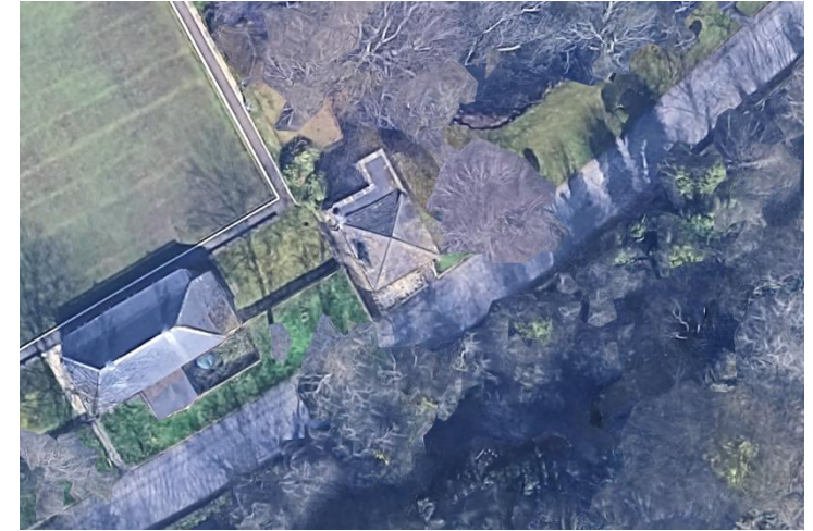
Satellite Imagery of existing building at 4 Brewery Drive (Google Maps, 2025)
