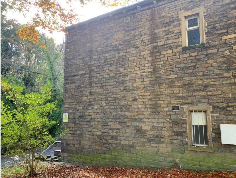
Photo 01 – External partial view of existing Side 1 Elevation (south side)
