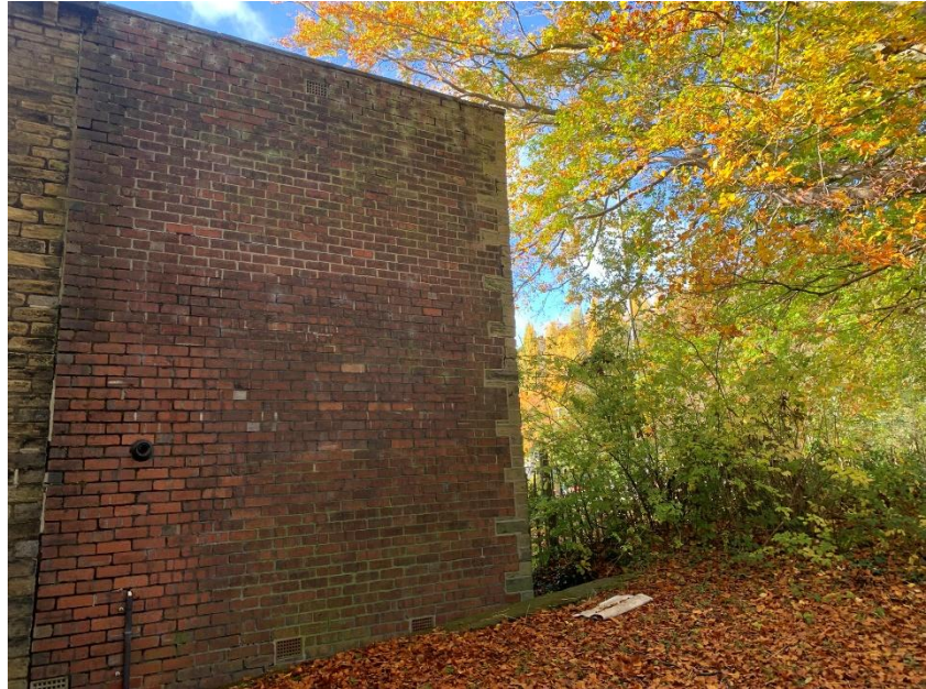
Photo 02 – External partial view of existing Side 1 Elevation (north side)
