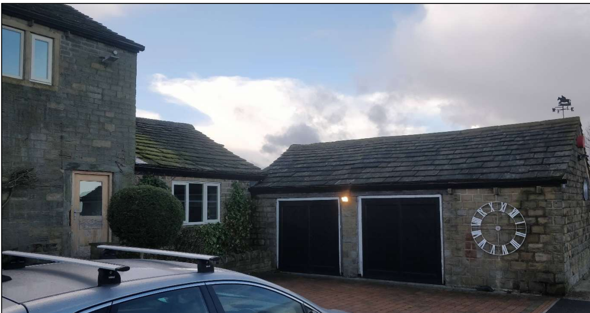
Existing tack room from the front/east
