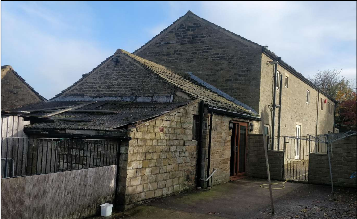
Existing tack room and lean-to extension from the north/west
