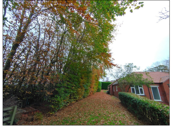
Photo 2: G9 running along the site's western boundary, looking north.
