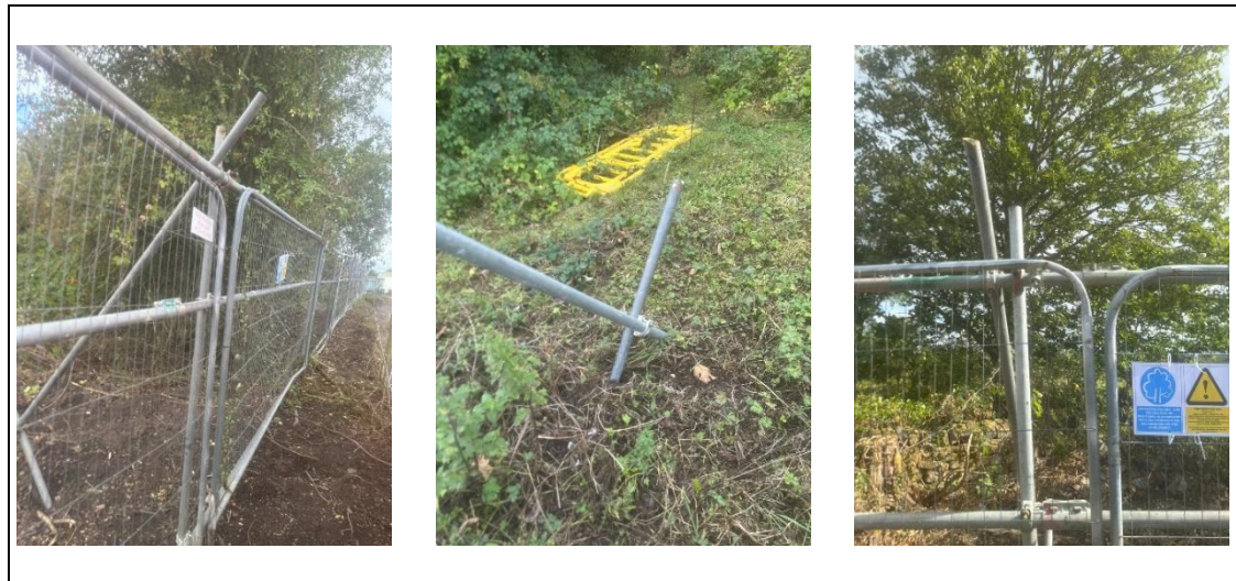
Figure 4.2: Examples of scaffold framework temporary tree protection fencing.
