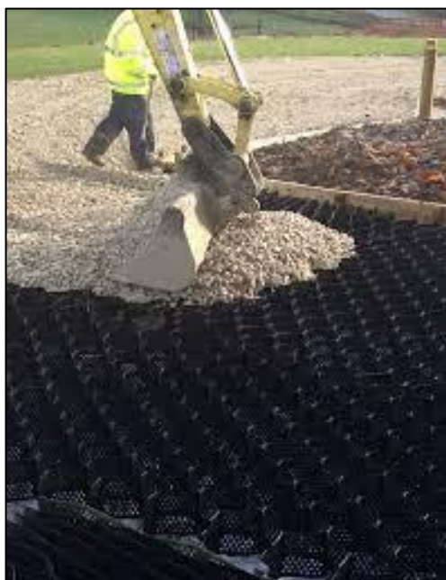
Figure 4.5: Cellweb® geo-cellular confinement sheets being infilled with 4/20 mm clean, angular stone.
