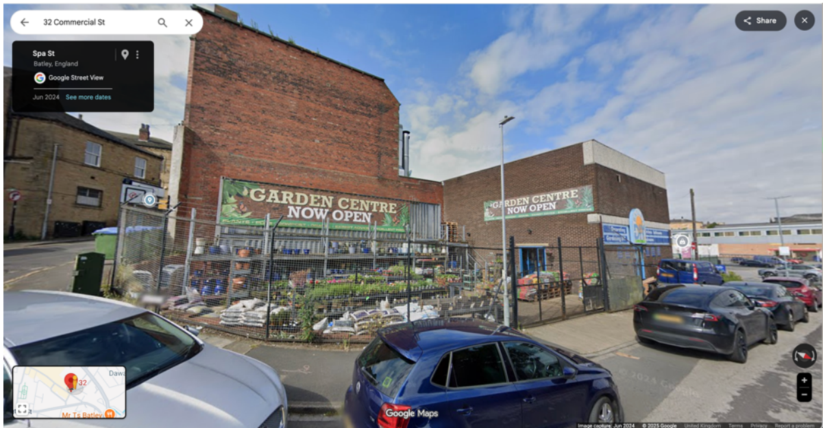
Application Site: Rear Elevation
