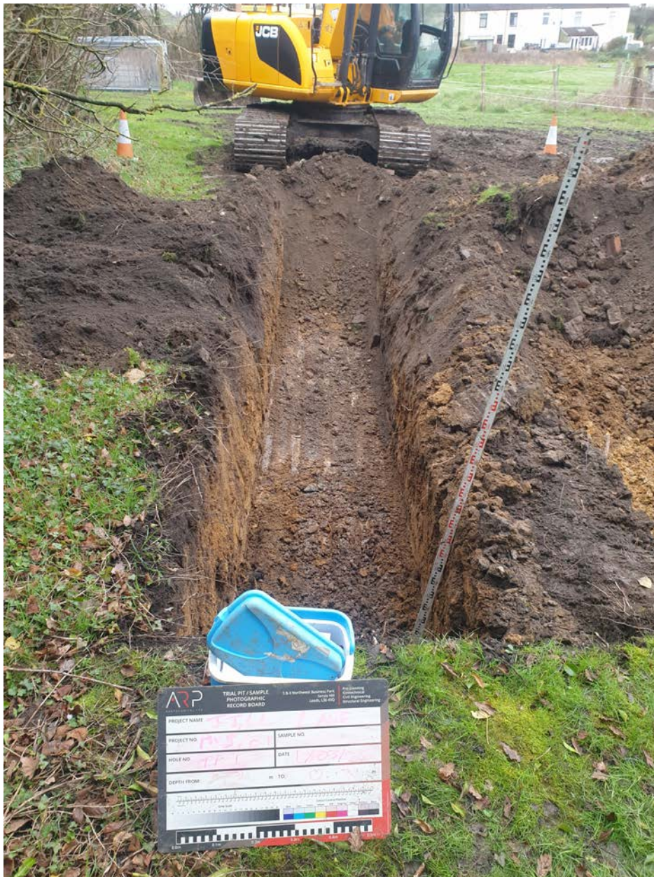
Photograph 1: Looking north, from southern boundary, shaft scrape excavated to rockhead.
