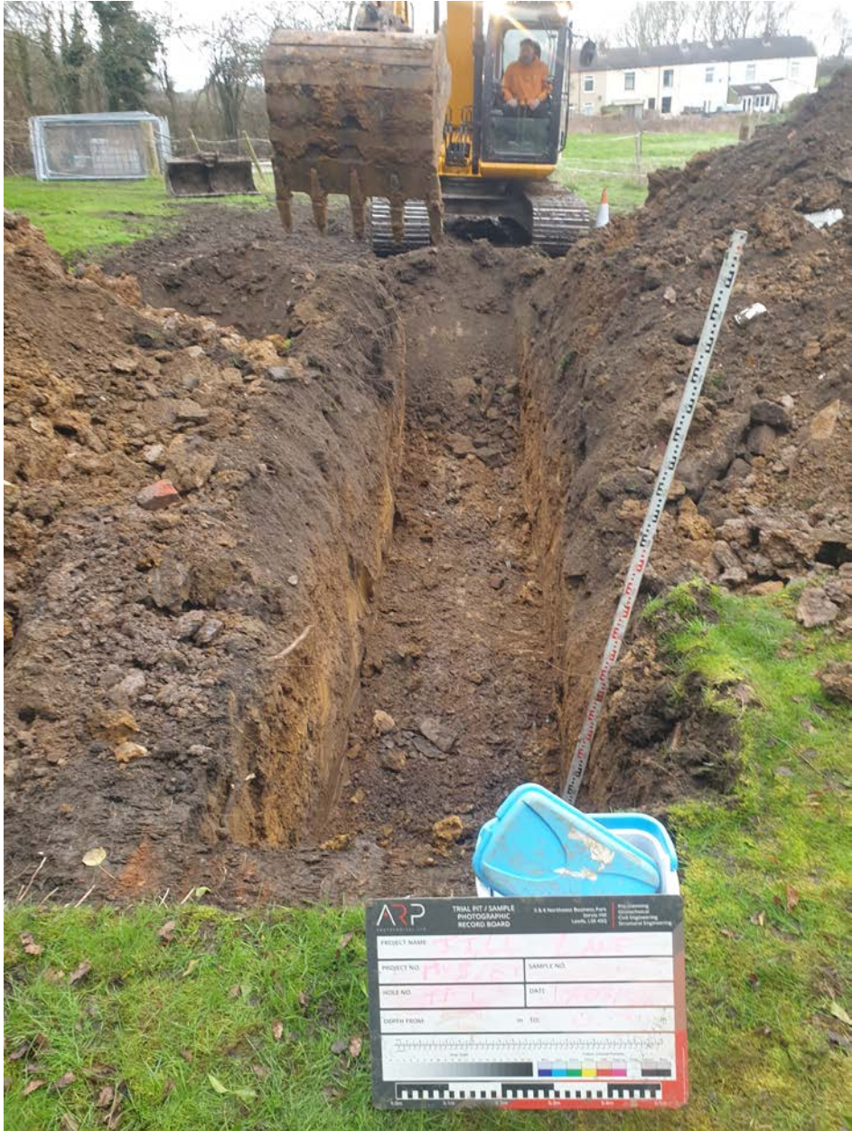
Photograph 2: Looking north, from southern boundary, shaft scrape excavated to rockhead.
