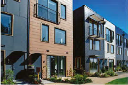
An example of energy efficient homes that are built off-site at the Climate Innovation District, Leeds (image: CITU)
