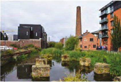
Combining industrial heritage and modern construction methods to create low carbon homes at Little Kelvin, Sheffield (image: FlickrAcademy of Urbanism)
