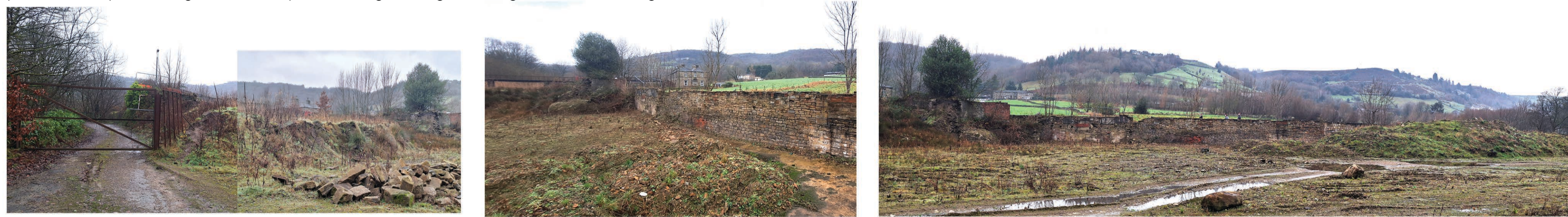
photos from site looking to site access road & entrance & towpath wall
