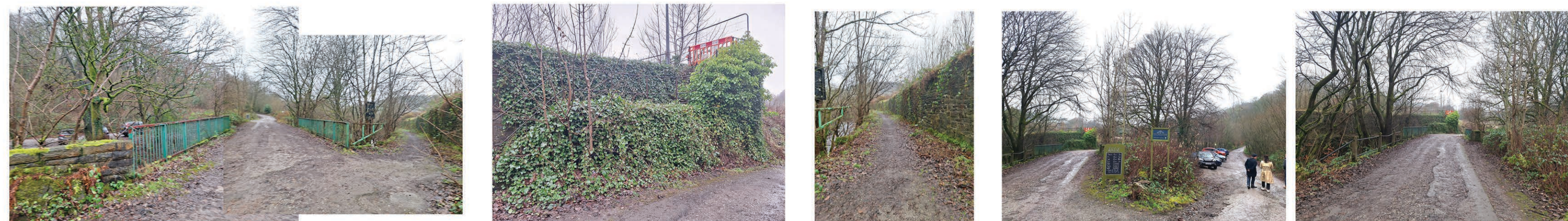
photos to site access road & bridge off manchester road & approach to site entrance & riverside access
