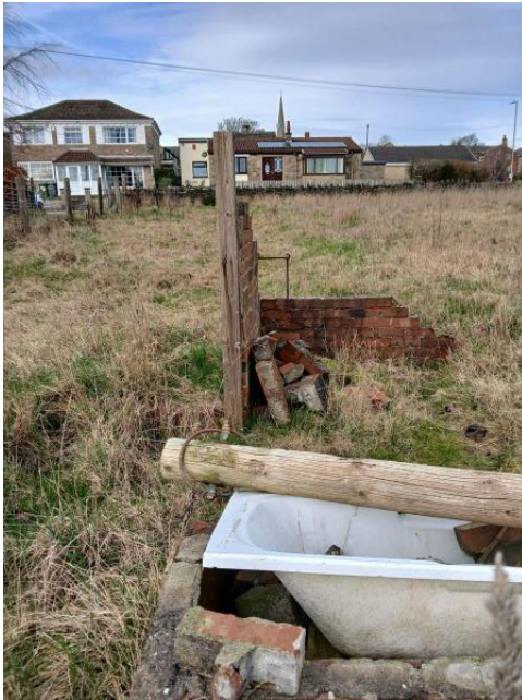
Photo 5: Remnants of walls found centrally on site.
