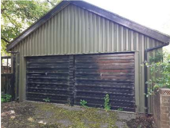
Photograph 5: Building B1, northern aspect (09.06.2022).
