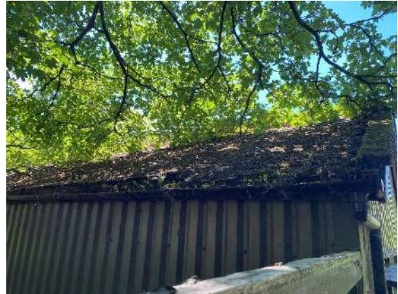
Photograph 6: Eastern roof pitch of Building B1 (07.07.2022).
