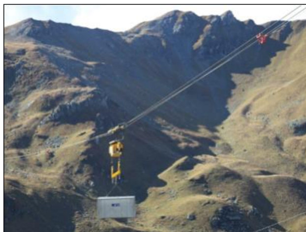
Figure 14: Typical cable crane
