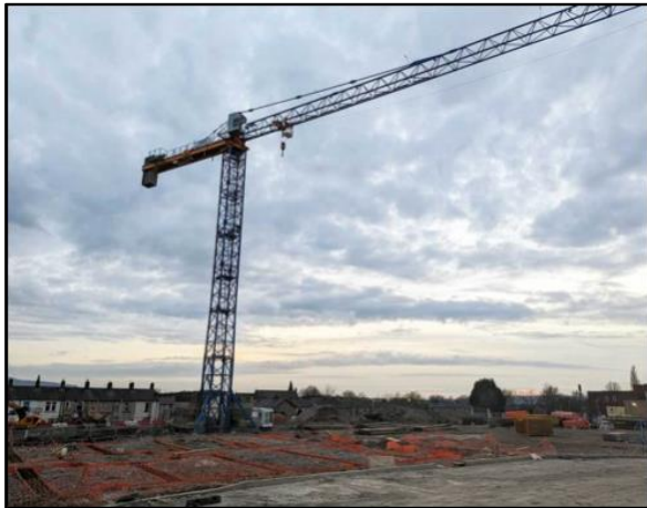
Figure 6 – Typical tower crane
