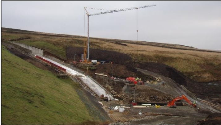
Figure 10 – Self-erecting tower crane spillway construction
