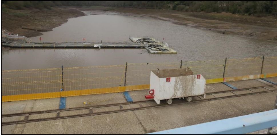
Figure 16: Narrow gauge rail system
