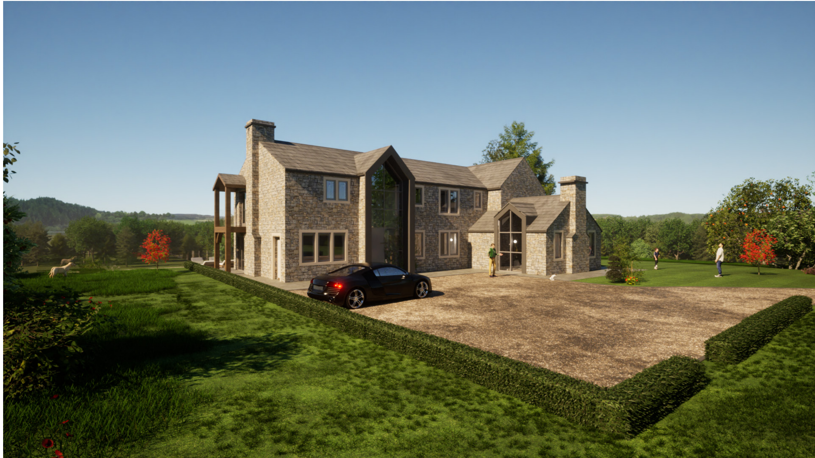
Proposed visualisation illustrating the view looking across the driveway / parking area to the southwest. A new double height glazed entrance highlights the new primary entrance, with a secondary entrance out of view on the southern elevation. A bronze anodised fascia will wraparound the projecting main entrance to juxtapose the monolithic natural stone and emphasise the main entrance.
