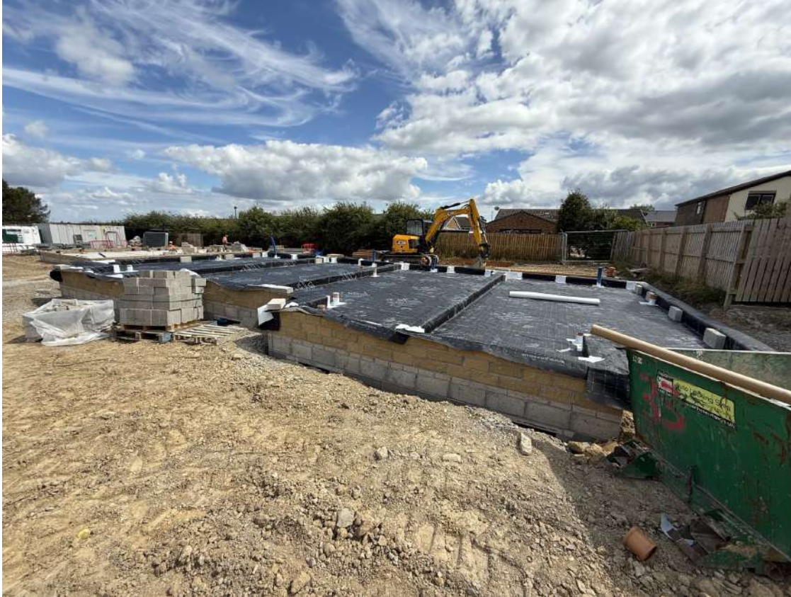
Plot 155-158 – Internal wall membrane layout with jointing
