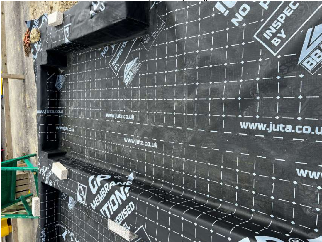
Plot 150-151 – Internal wall membrane layout with jointing
