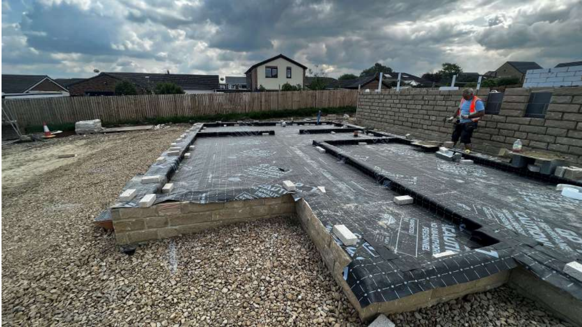
Plot 159 – Internal wall membrane layout with jointing
