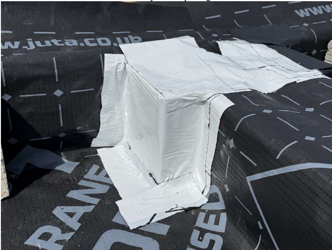
Plot 155-158 – Internal wall membrane layout with jointing
