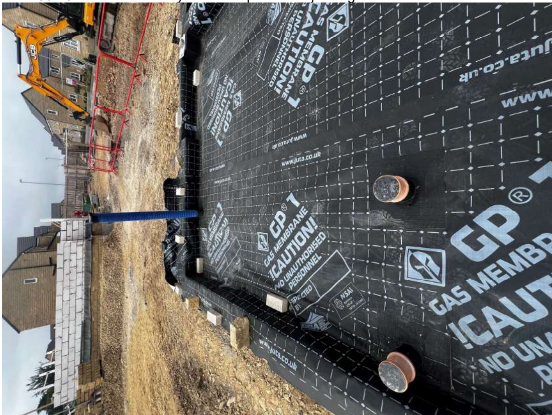
Plot 150-151 – Membrane layout with tophats and jointing
