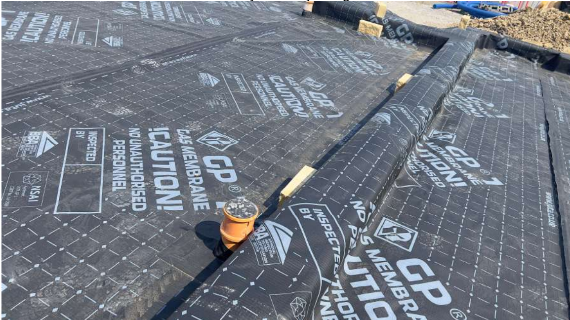
Plot 152-154 – Internal wall membrane layout with jointing
