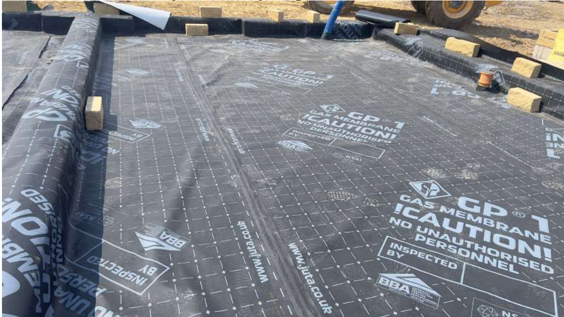
Plot 152-154 – Membrane layout with tophats and jointing
