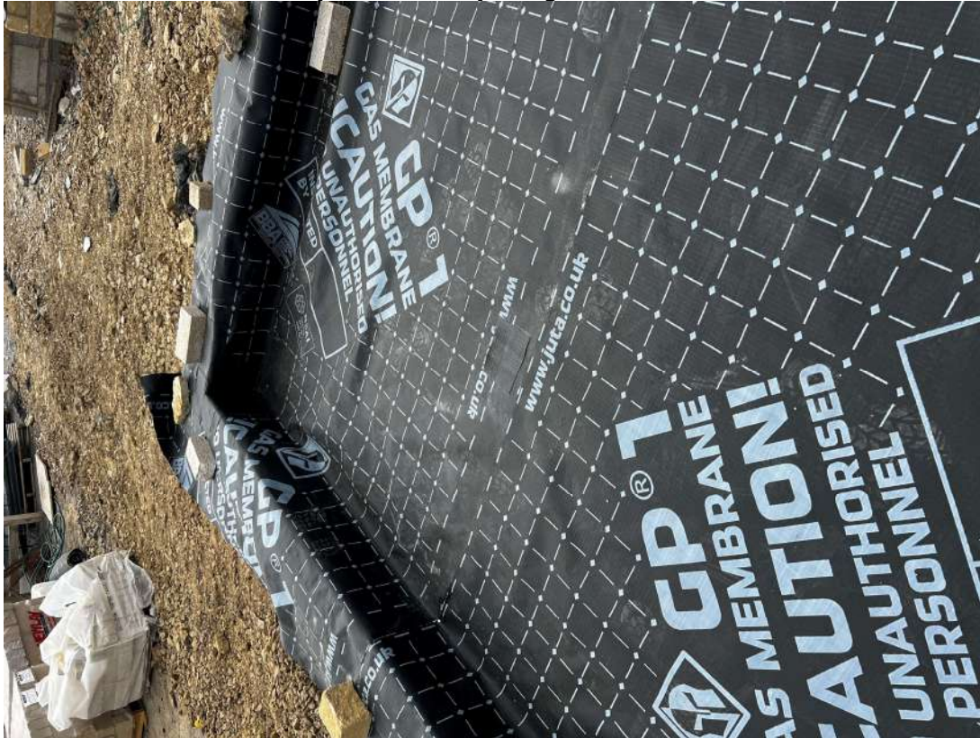
Plot 150-151 – Membrane layout with tophats and jointing
