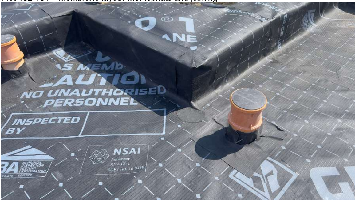
Plot 152-154 – Membrane layout with tophats and jointing
