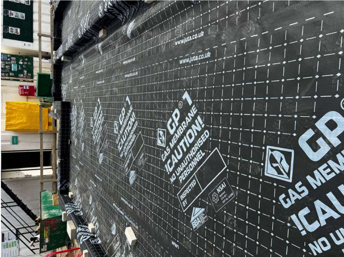
Plot 150-151 – Internal wall membrane layout with jointing
