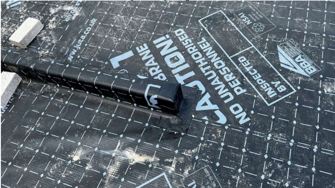
Plot 159 – Internal wall membrane layout with jointing
