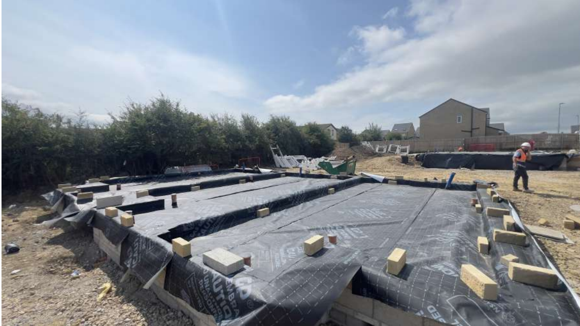
Plot 152-154 – Internal wall membrane layout with jointing
