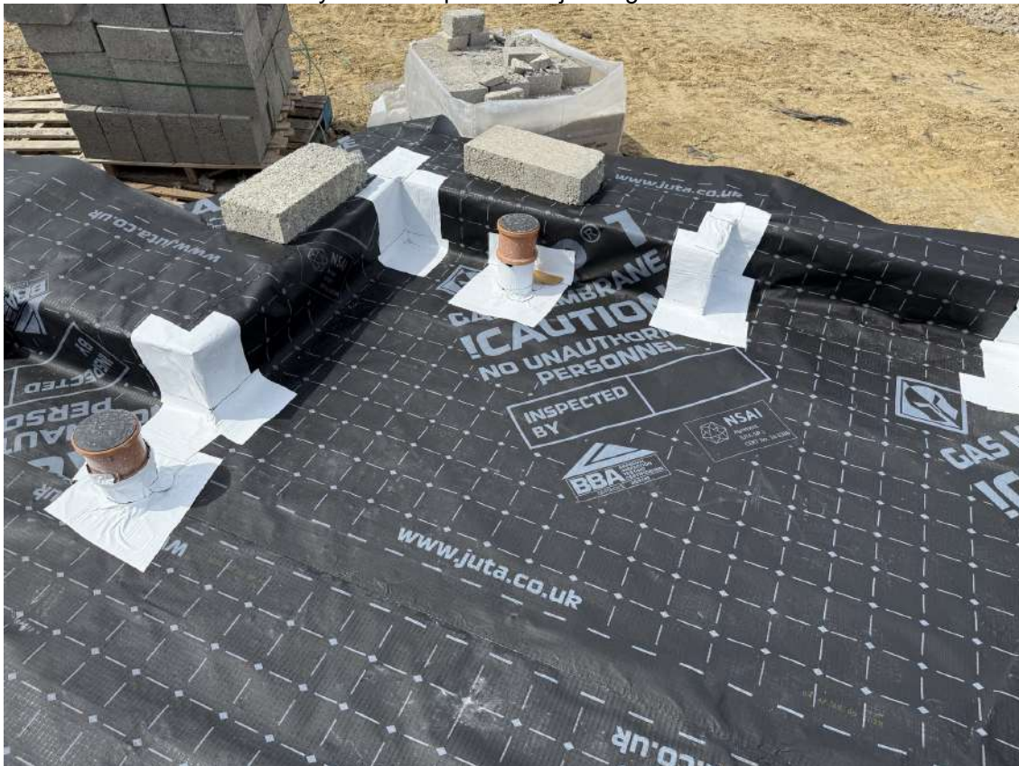
Plot 155-158 – Membrane layout with tophats and jointing
