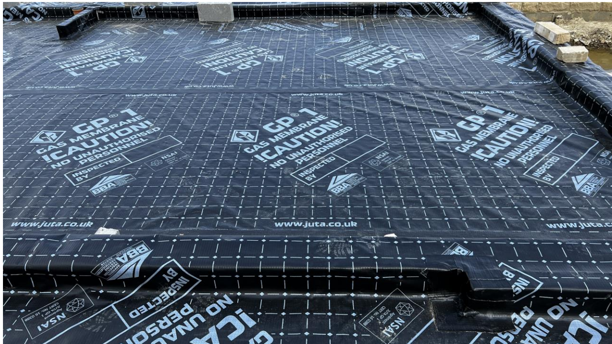
Plot 89 – Membrane layout with tophat and jointing
