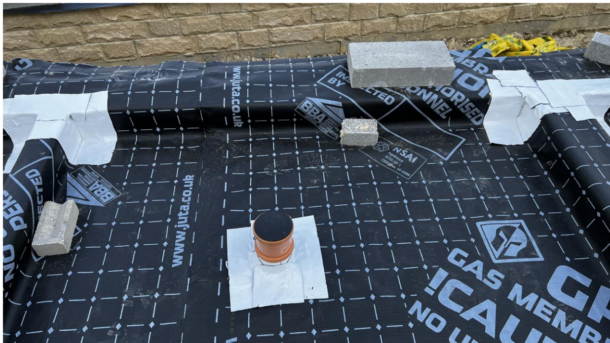
Plot 89 – Membrane layout with tophat and jointing
