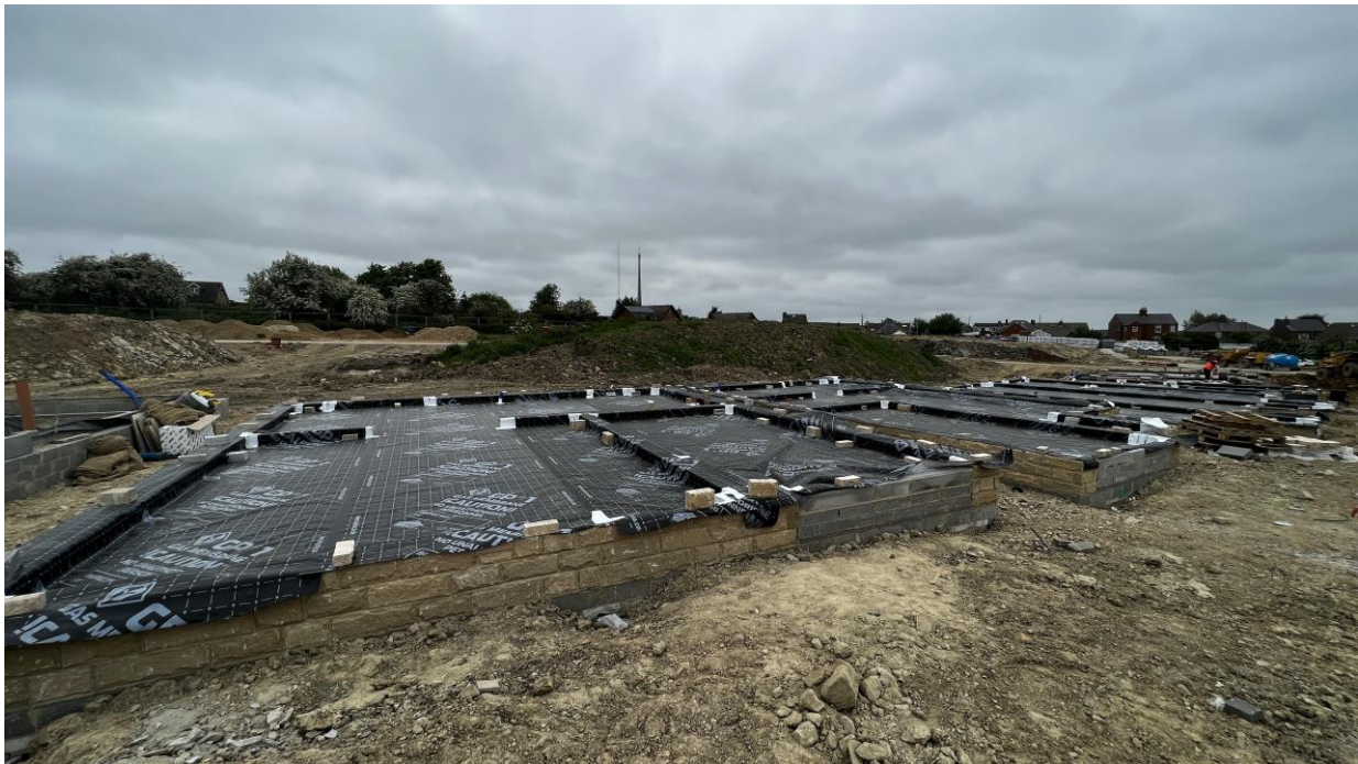
Plot 83 – Membrane layout with weld joint and internal walls.
