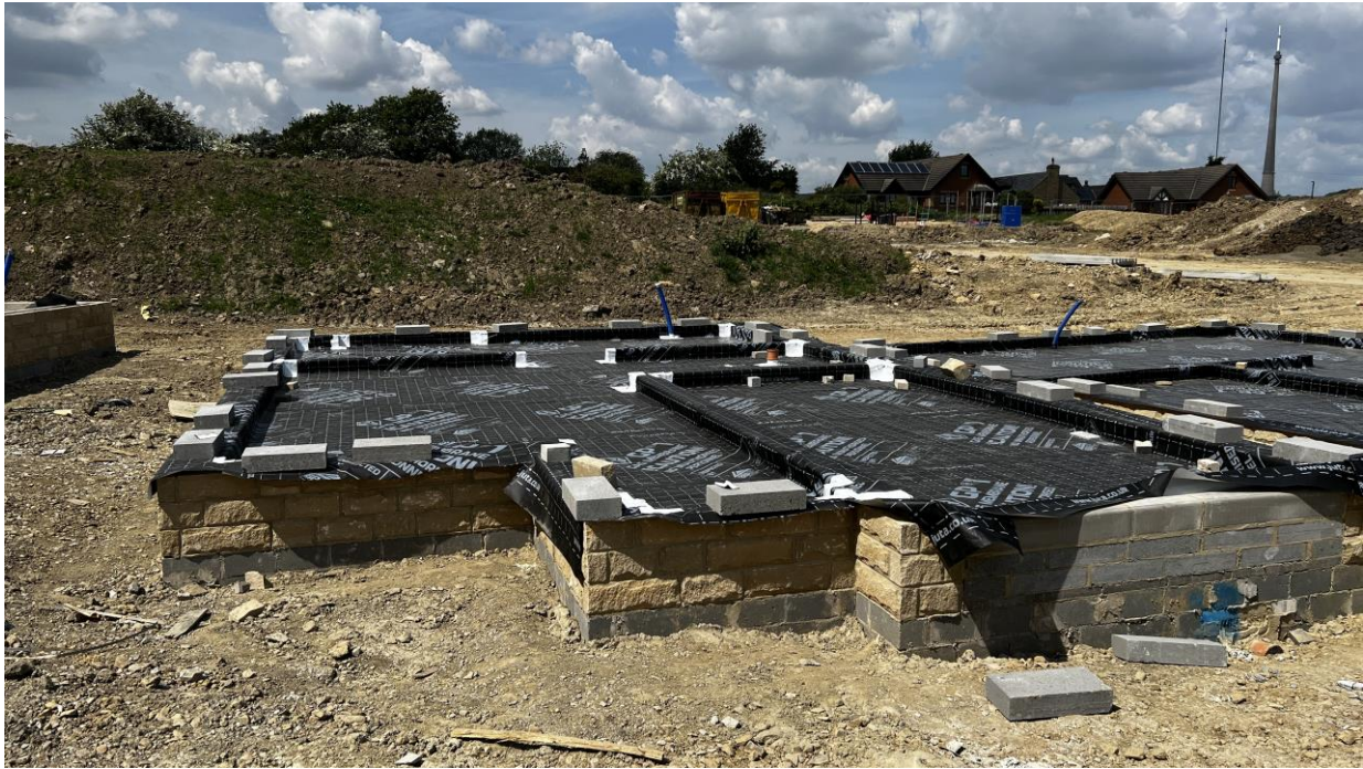
Plot 88 – Membrane layout with tophat and jointing
