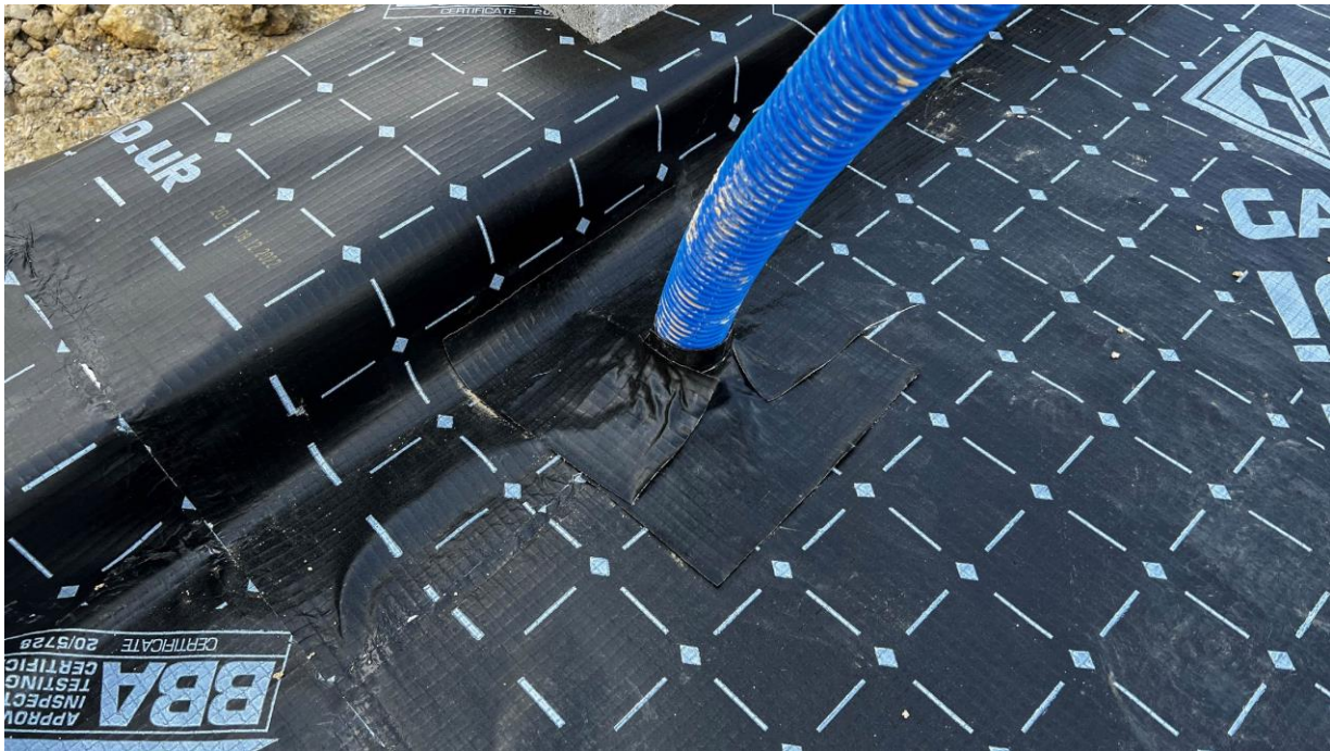
Plot 88 – Membrane layout with tophat and jointing
