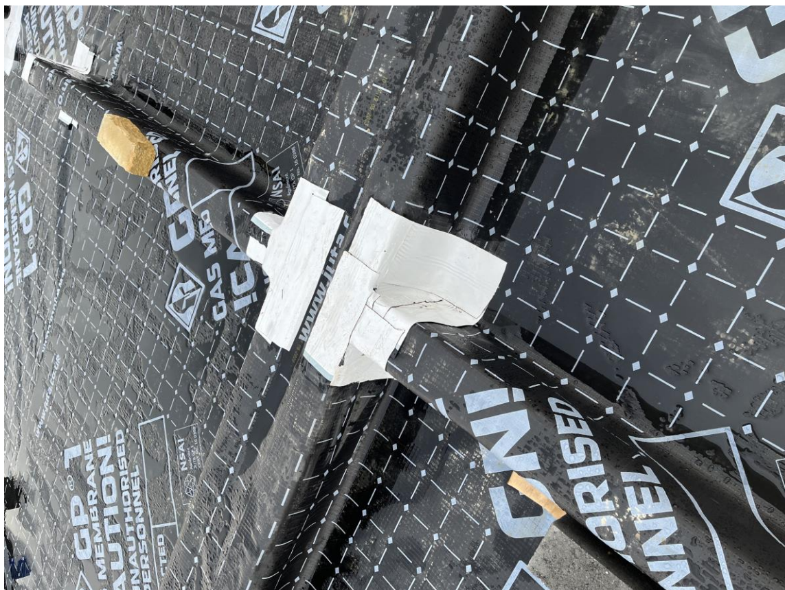
Plots 133 & 134 – Party wall membrane layout with jointing
