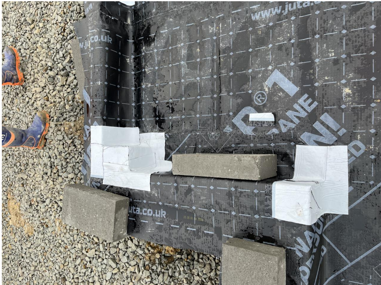
Plot 135 - Membrane layout with jointing
