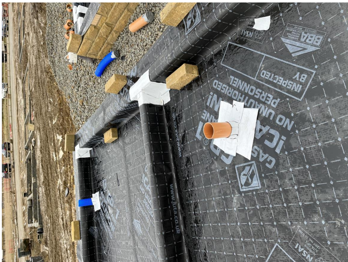
Plot 129 - Membrane layout with tophat and jointing
