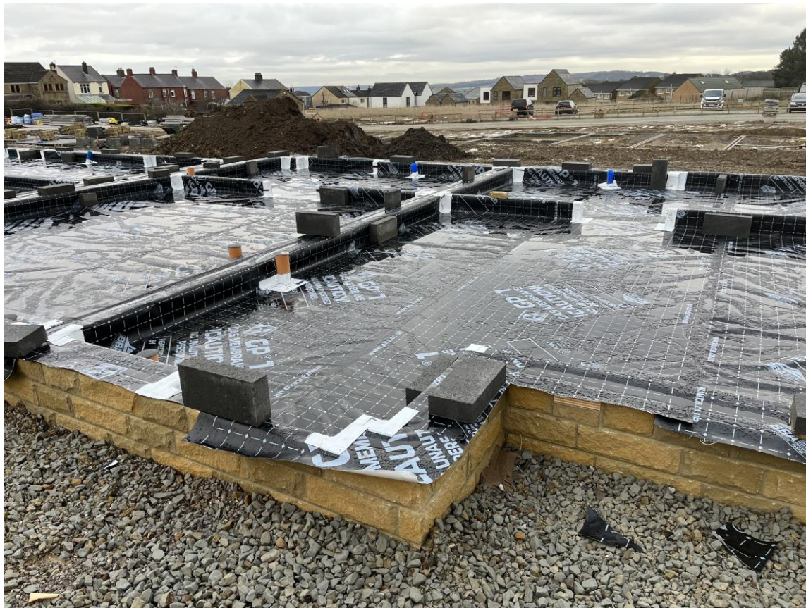
Plots 133 & 134 – Party wall membrane layout with jointing
