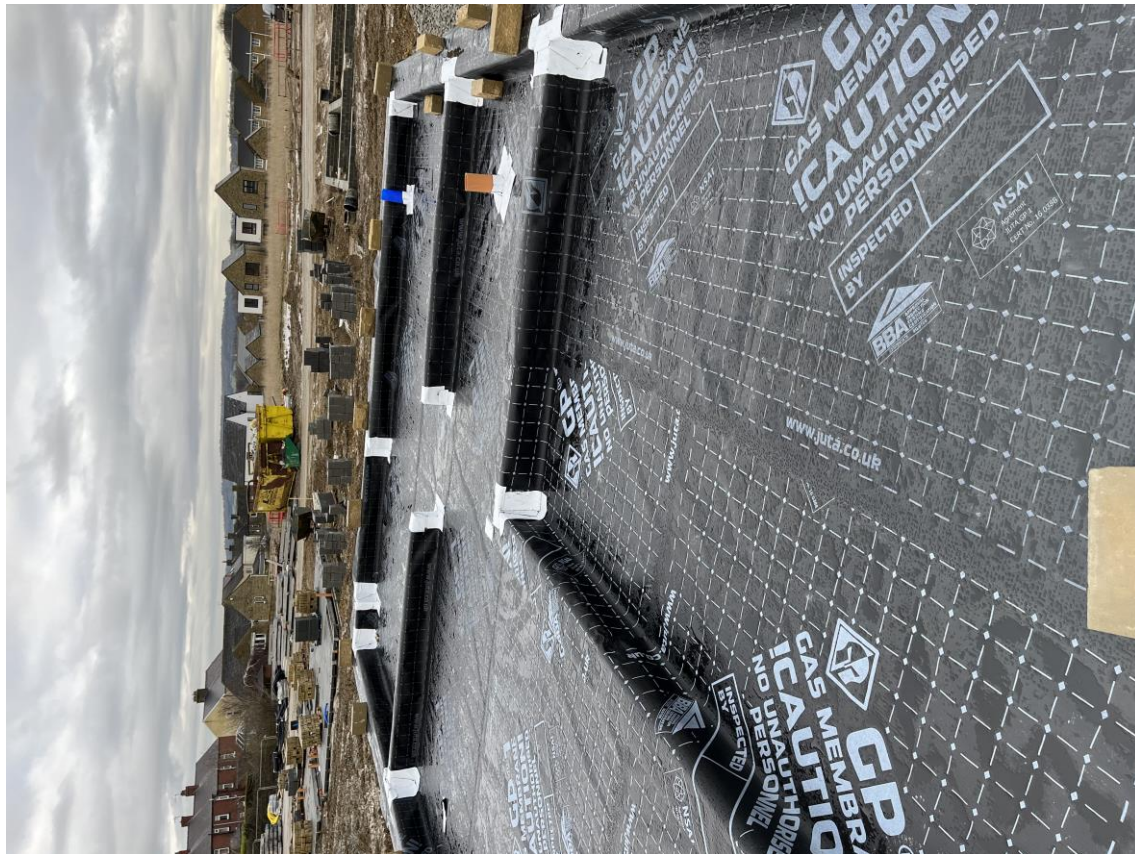
Plot 129 - Membrane layout with tophat and jointing
