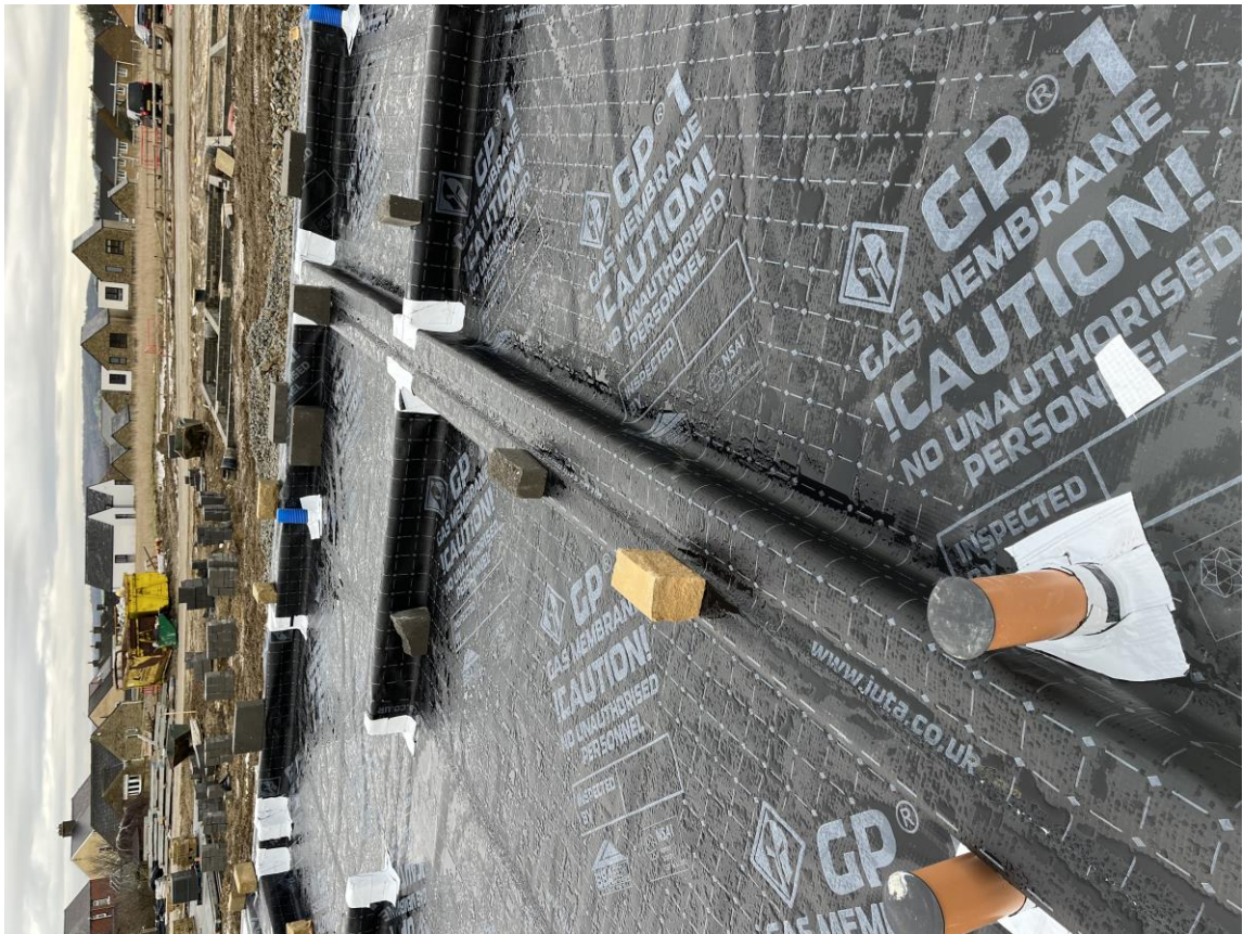
Plots 130 & 131 – Overall membrane layout with party wall and tophat with jointing
