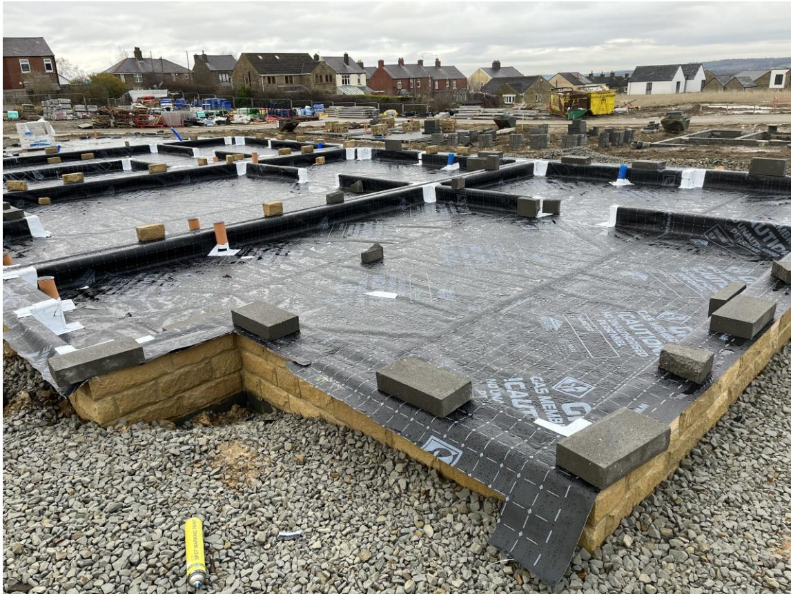
Plots 130 & 131 – Overall membrane layout with party wall and tophat with jointing
