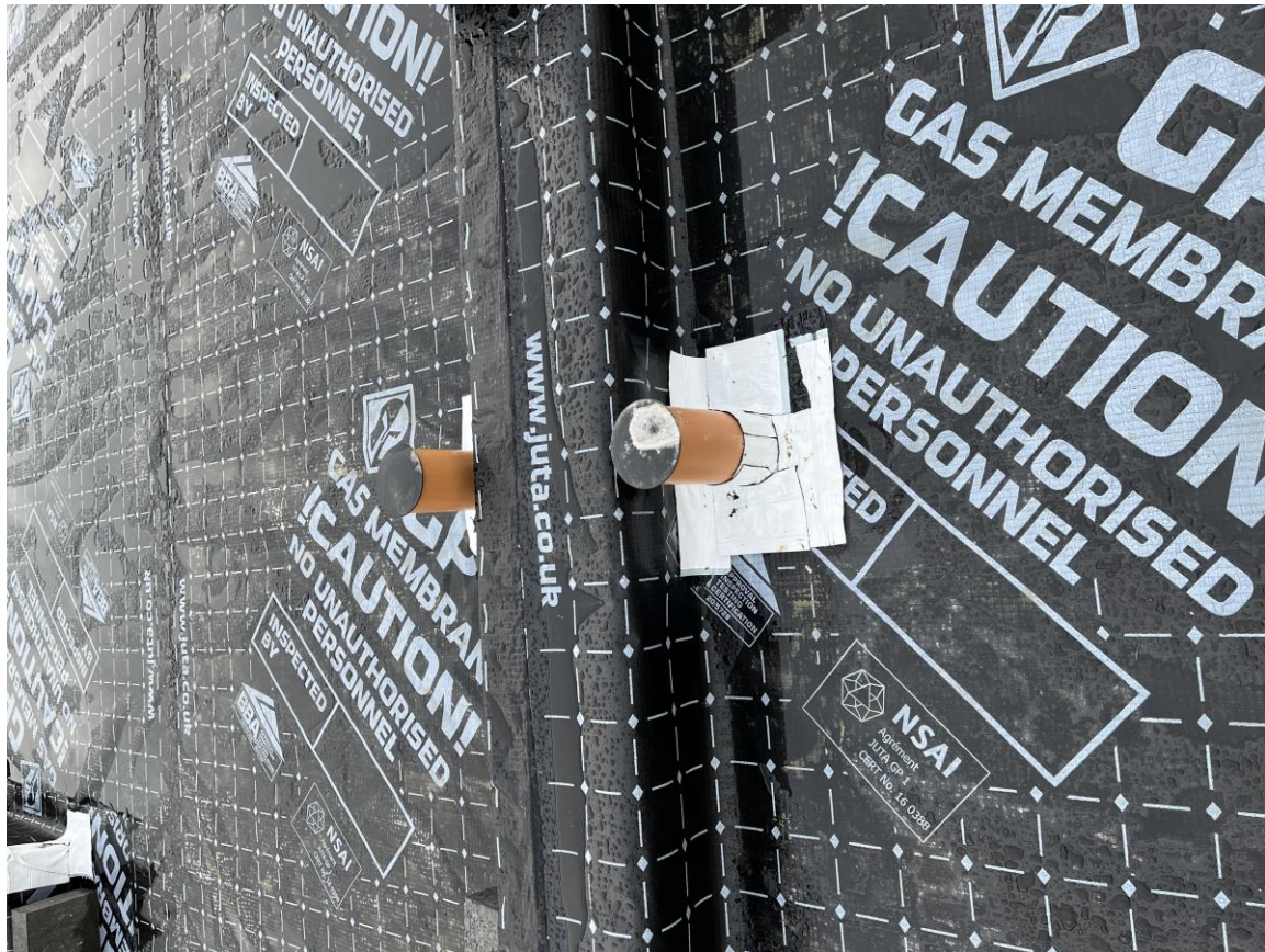
Plot 135 – Internal wall membrane layout with tophat and jointing
