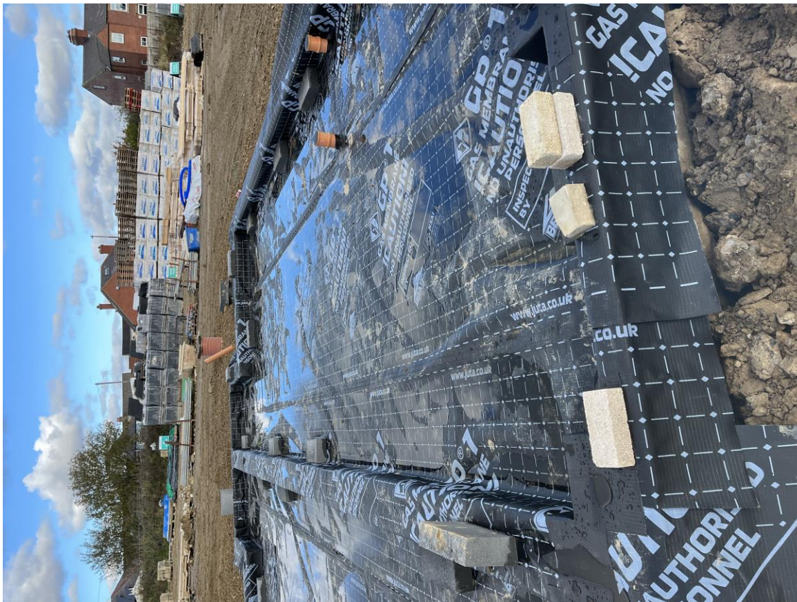
Plots 100 & 101 - Membrane layout with party wall and jointing
