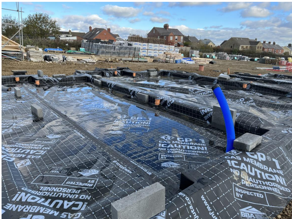
Plots 102-104 – Overall membrane layout with weld, party wall and tophats
