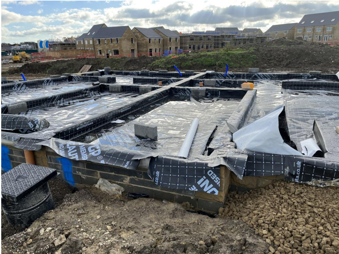
Plots 105 & 106 - Internal wall and party wall membrane layout with jointing
