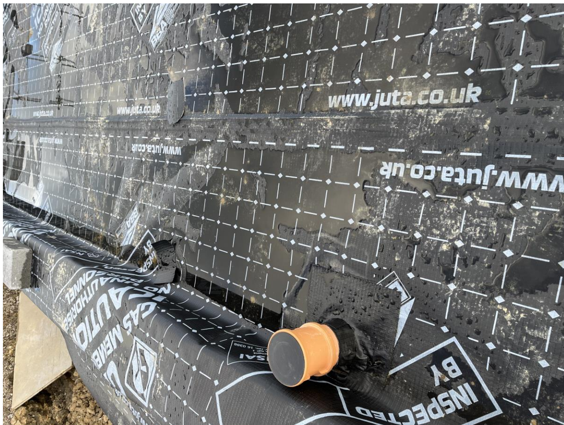
Plots 102-104 – Membrane layout with weld and tophat with jointing
