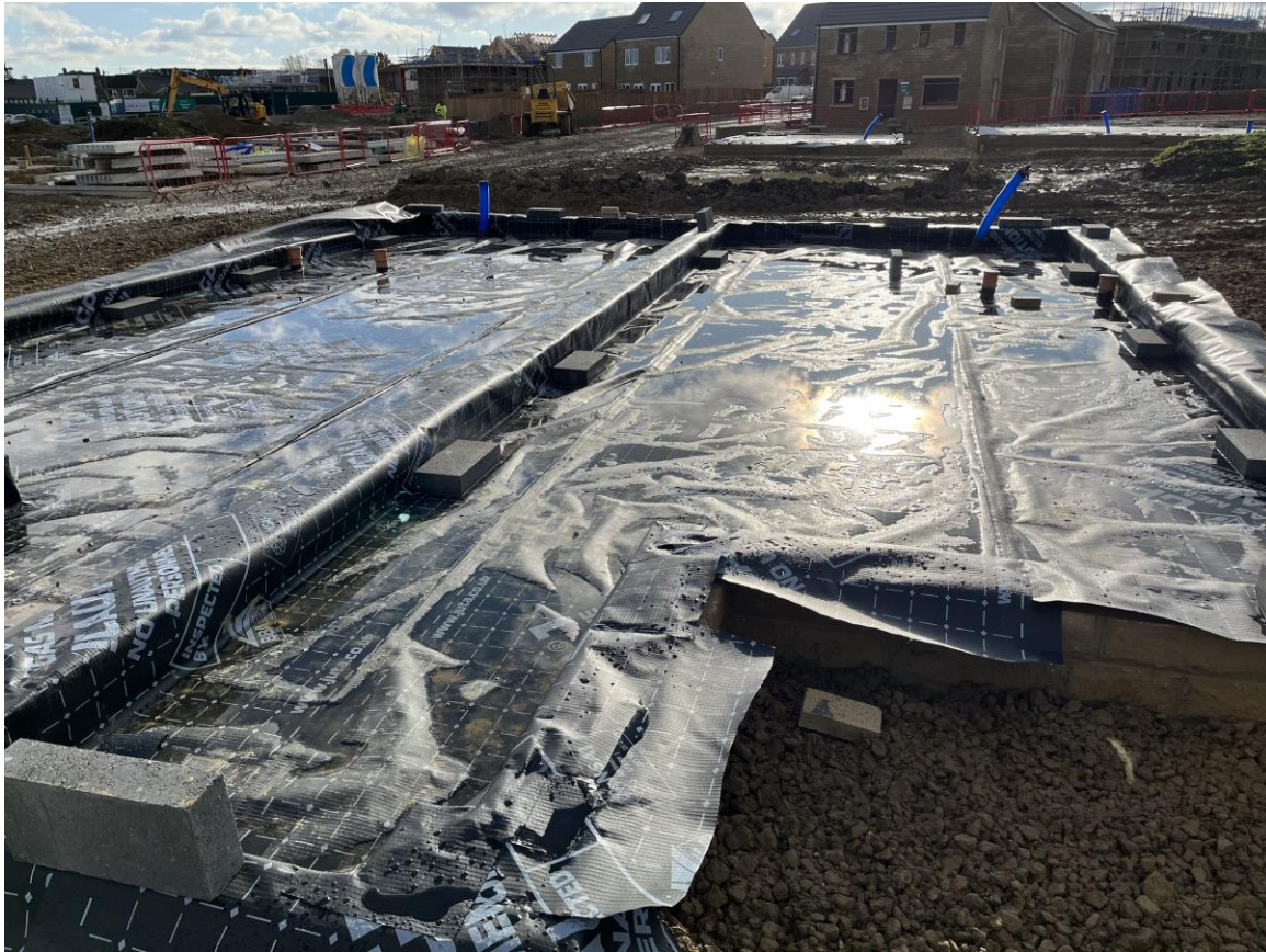
Plots 100 & 101 - Membrane layout with party wall and jointing
