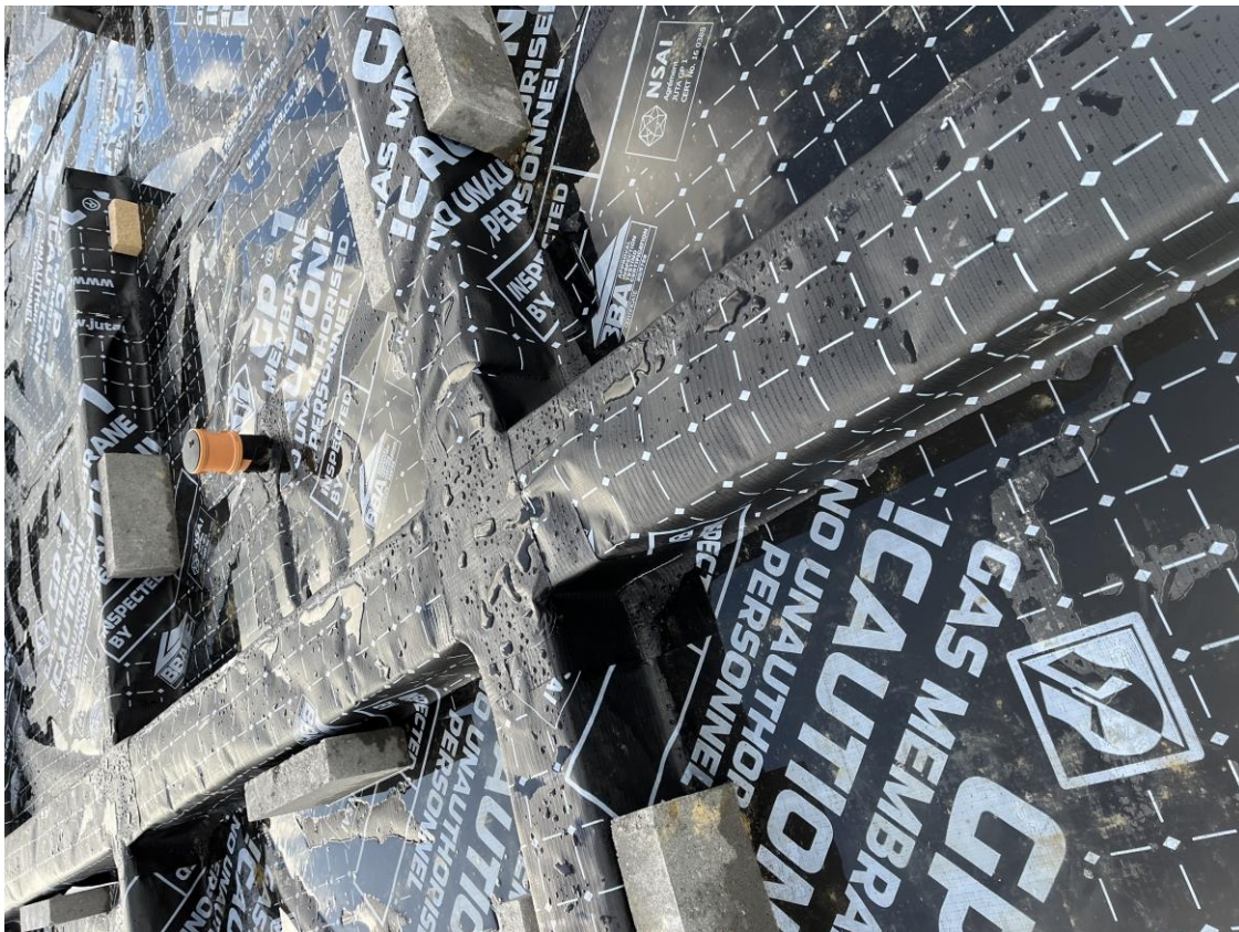
Plots 105 & 106 - Internal wall and party wall membrane layout with jointing
