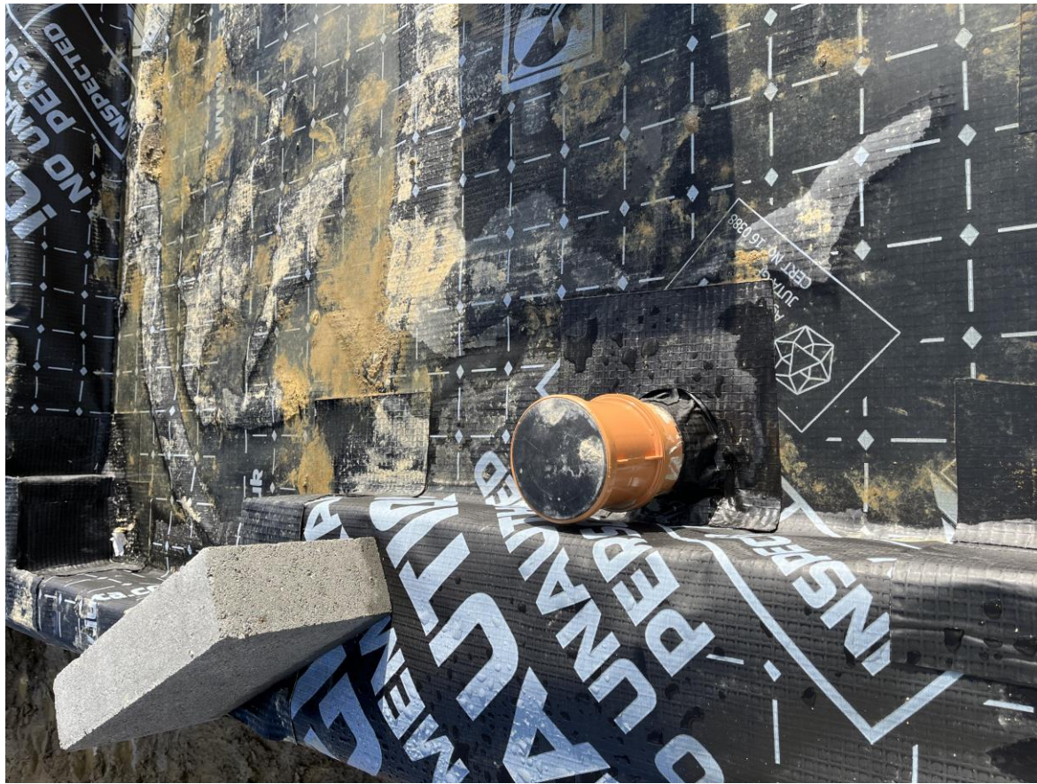
Plots 125 & 126 – Membrane layout with welds
