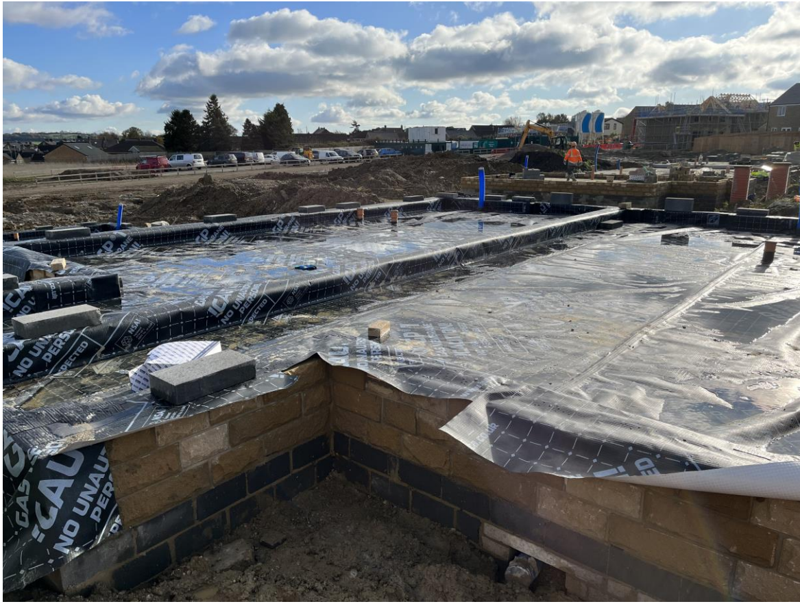
Plots 127 & 128 – Membrane layout with tophat and jointing
