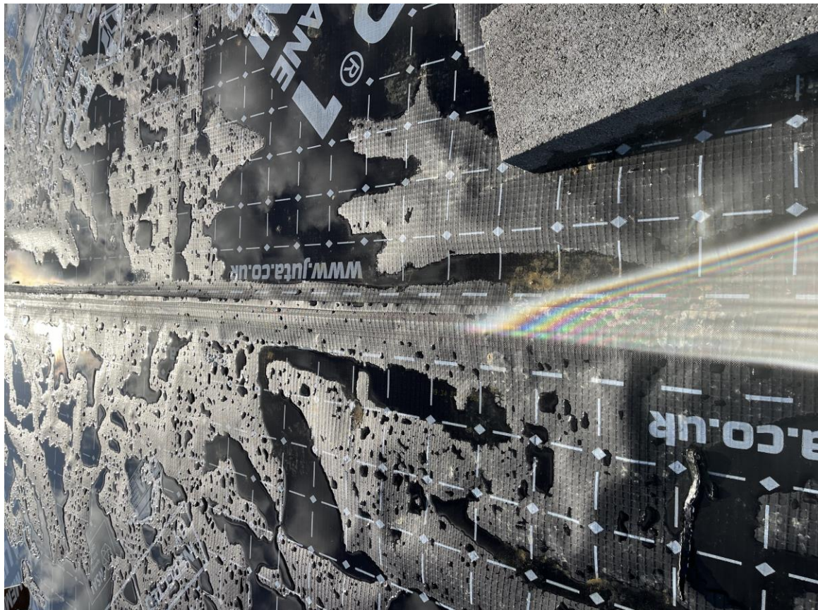
Plots 125 & 126 – Membrane layout with welds
