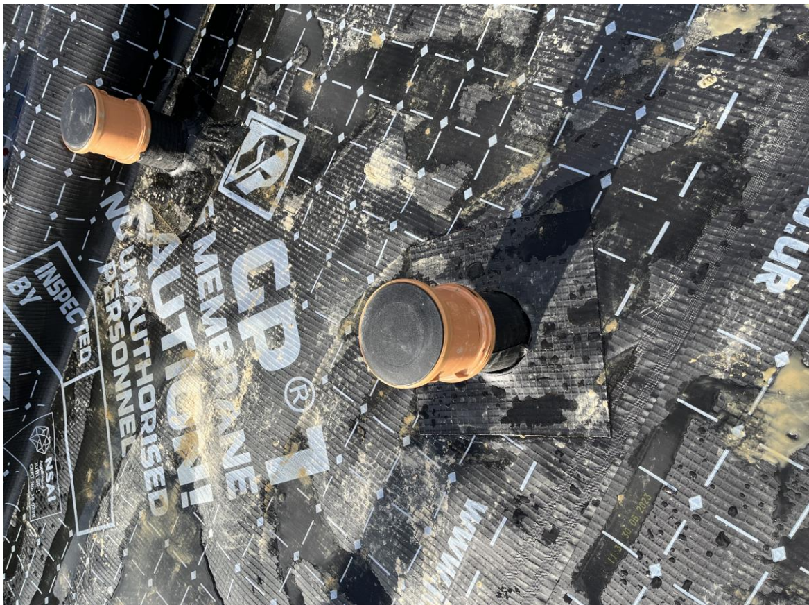
Plots 127 & 128 – Membrane layout with tophat and jointing
