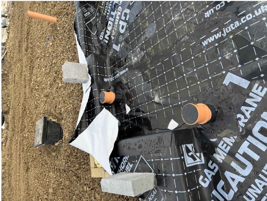
Plots 102-104 – Membrane layout with weld and tophat with jointing
