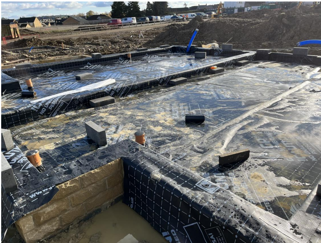
Plots 125 & 126 – Overall membrane layout
