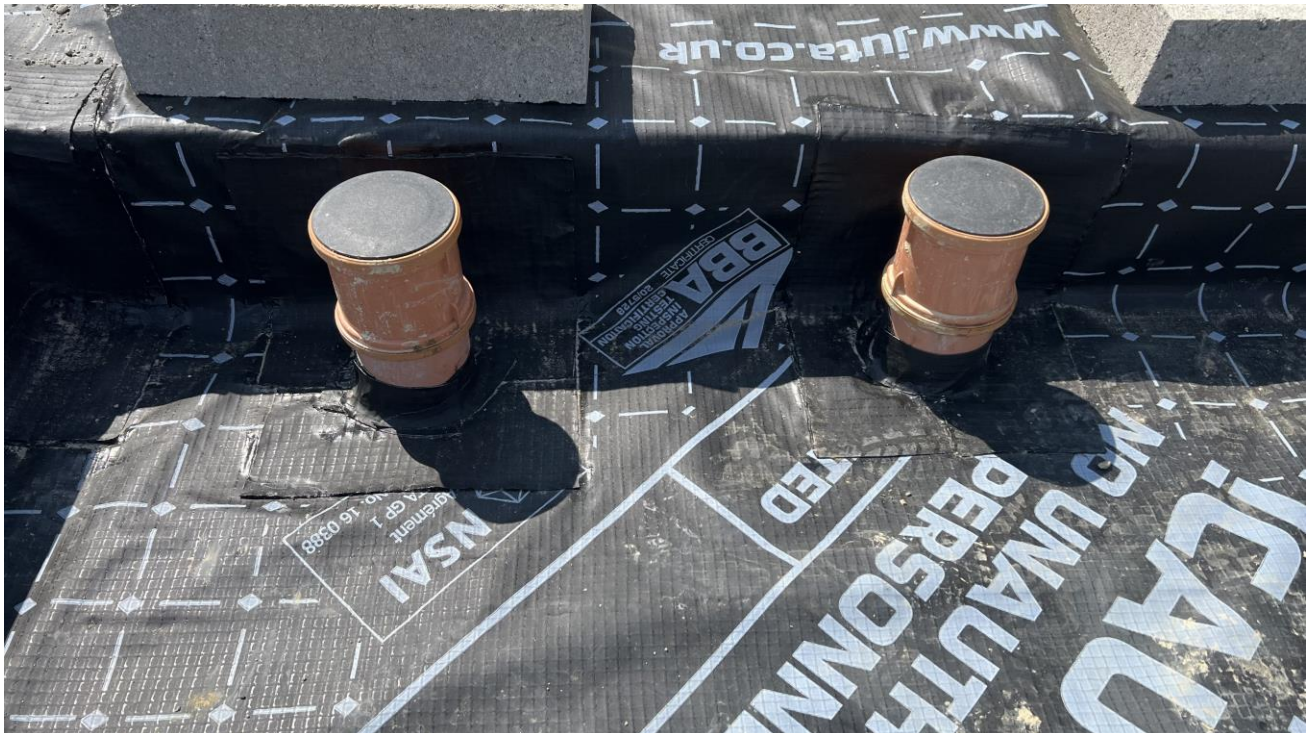
Plot 119 - Membrane layout with tophats and jointing
