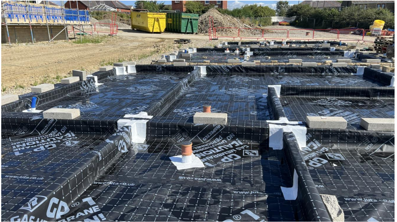
Plots 121 & 122 – Membrane layout with tophat and jointing
