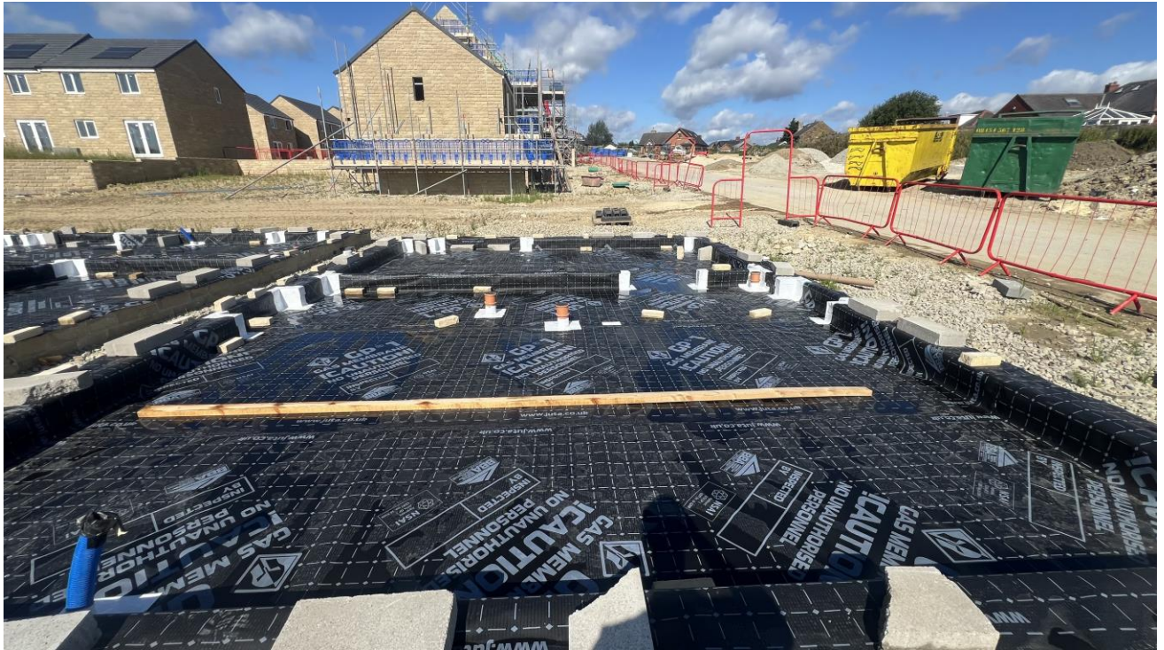
Plot 124 – Membrane layout with tophat and jointing
