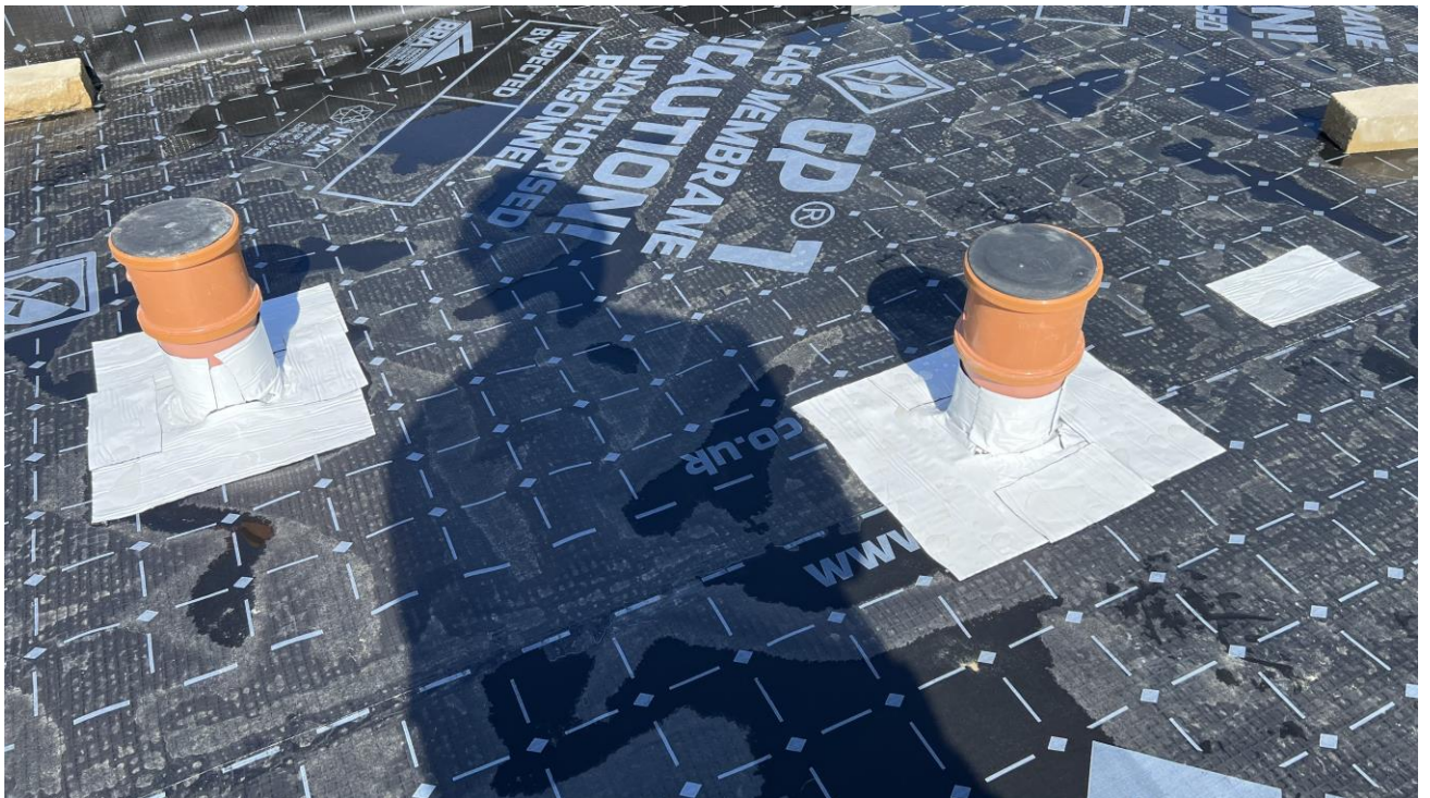
Plot 124 – Membrane layout with tophat and jointing
