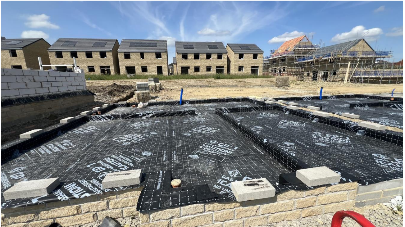
Plot 119 - Membrane layout with tophats and jointing
