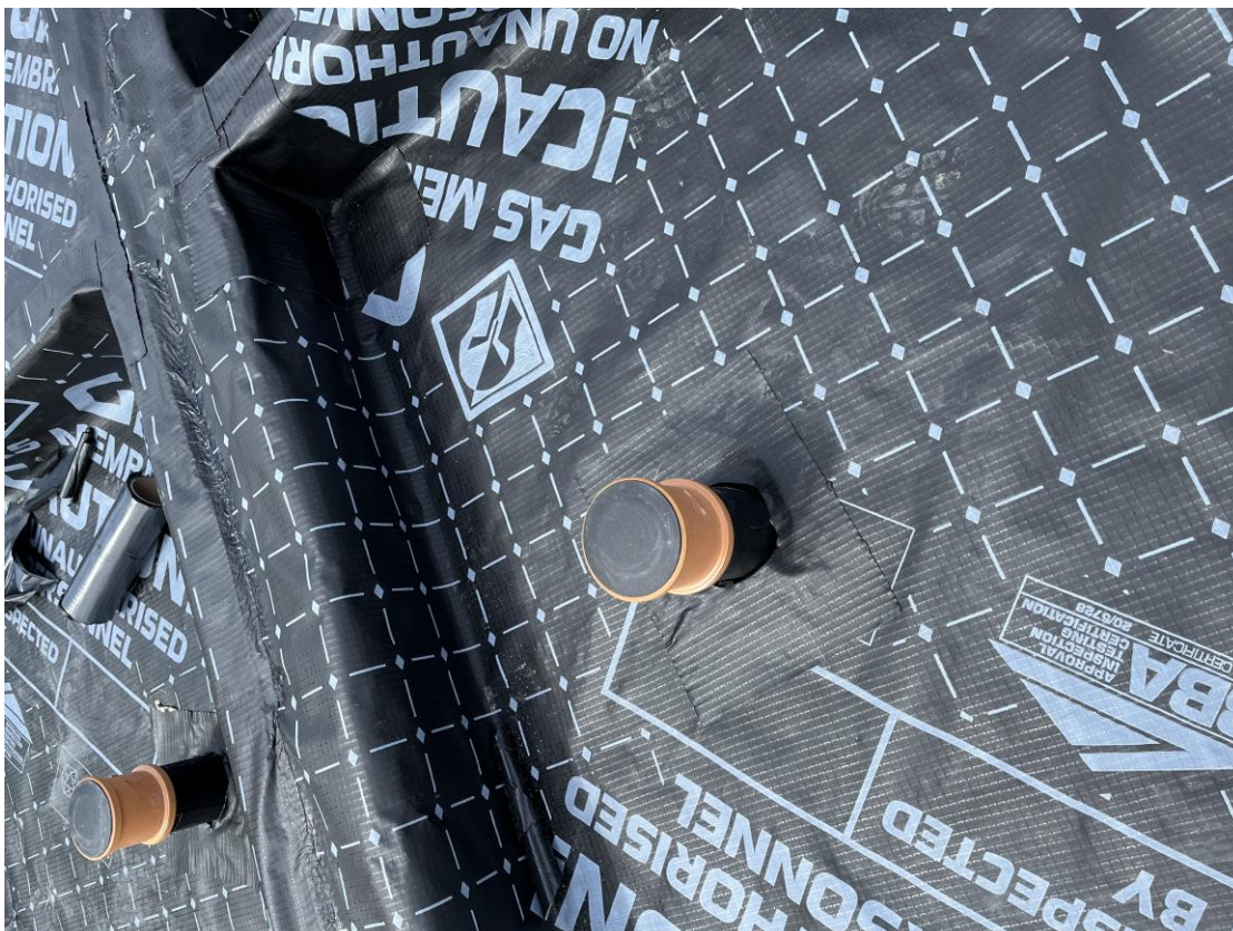
Plots 142 & 143 - Membrane layout with tophats, party wall and jointing
