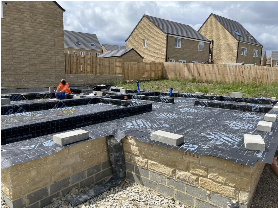
Plots 142 & 143 - Membrane layout with tophats, party wall and jointing
