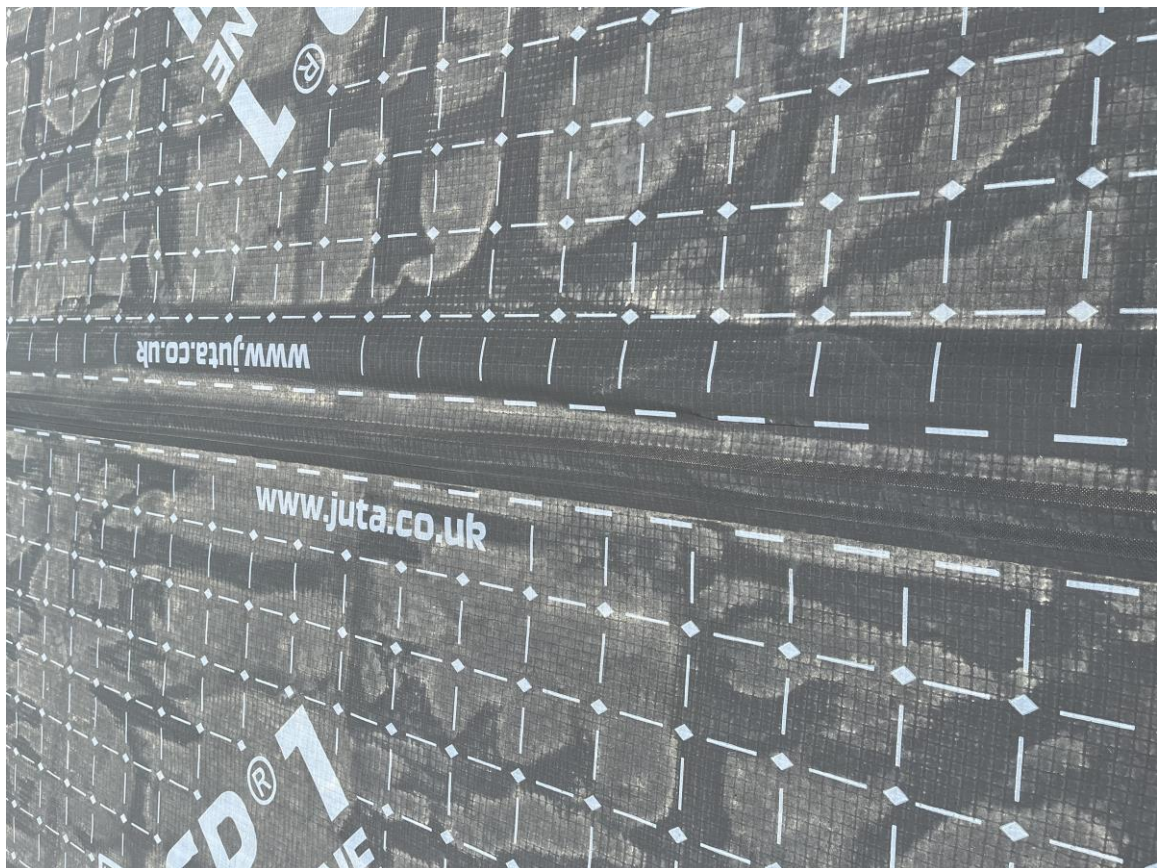
Plots 146-149 – Membrane layout with weld joint
