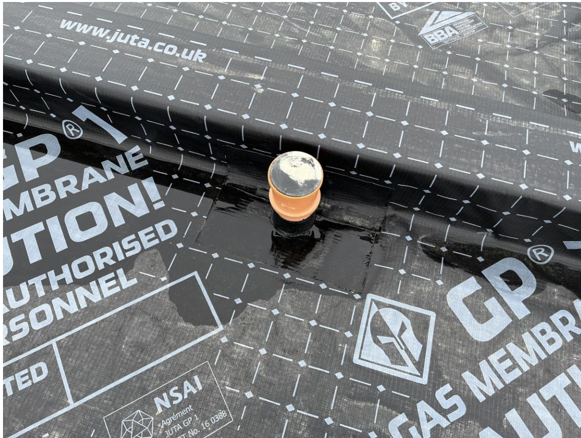
Plots 146-149 – Membrane layout with weld joint
