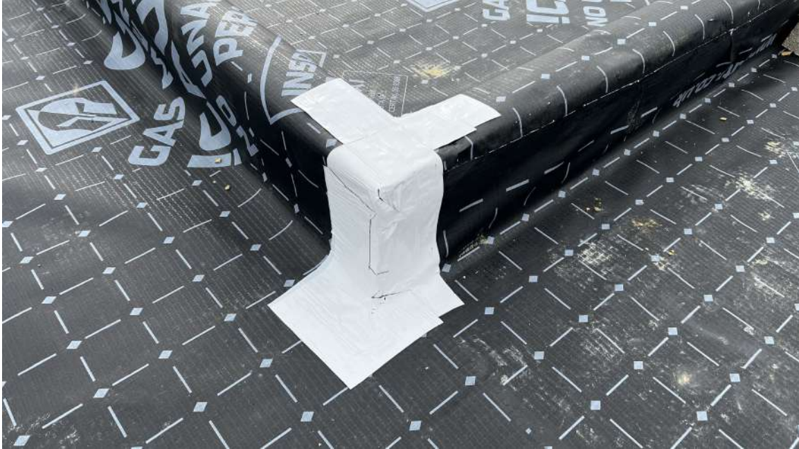
Plot 109 – Membrane layout with weld jointing
