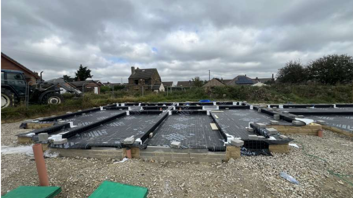
Plot 109 – Membrane layout with tophats and jointing
