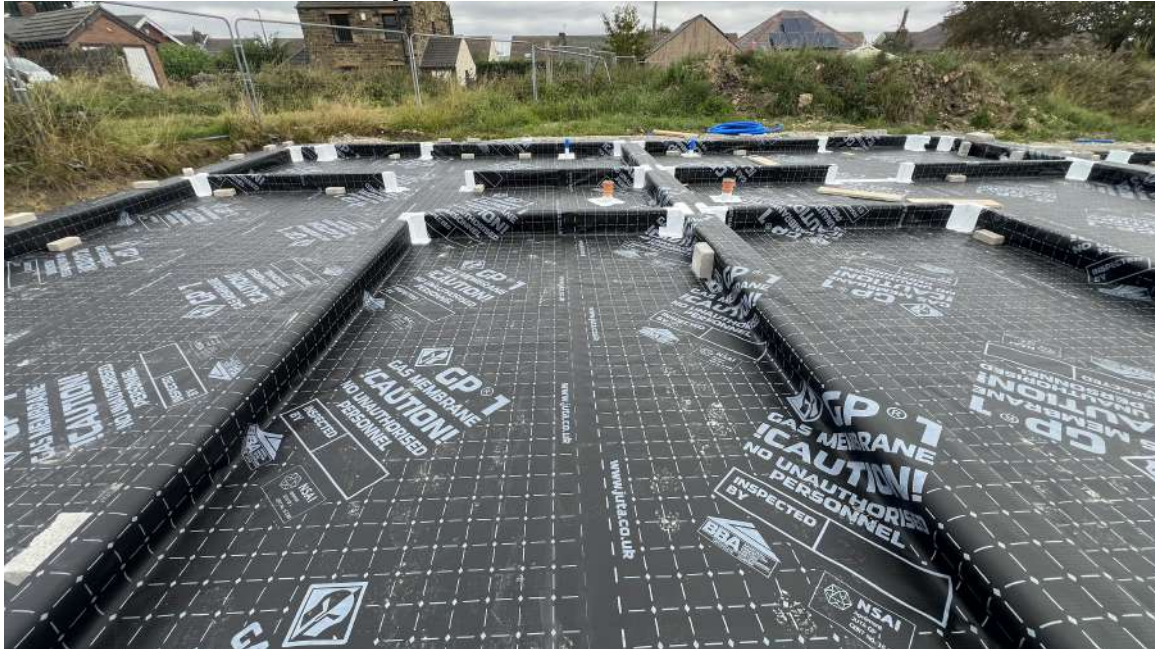
Plot 108 - Membrane layout with tophats and jointing
