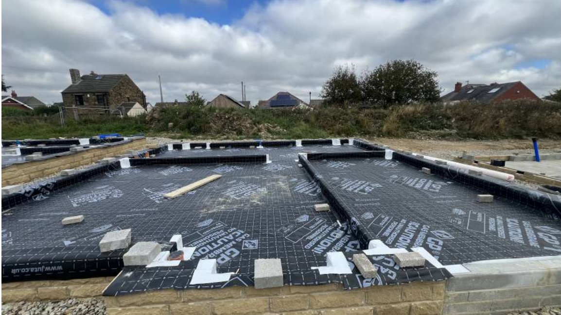
Plot 110 – Membrane layout with internal wall and jointing
