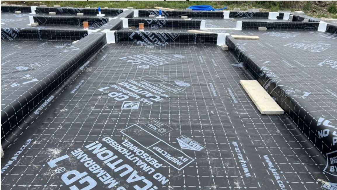
Plot 109 – Membrane layout with tophats and jointing
