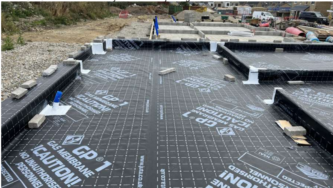
Plot 110 – Overall membrane layout with weld jointing
