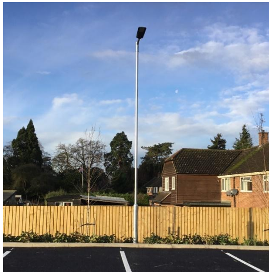
Fig 8: External LED Lighting.
