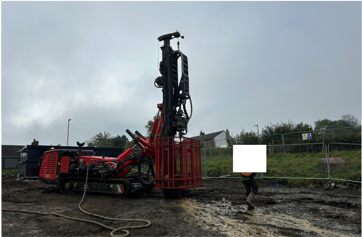
Photograph 1 – Drill and Grout works
