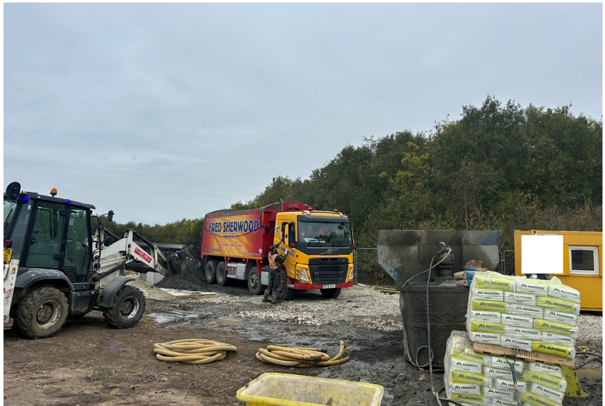
Photograph 2 – Photograph during the delivery of PFA.
