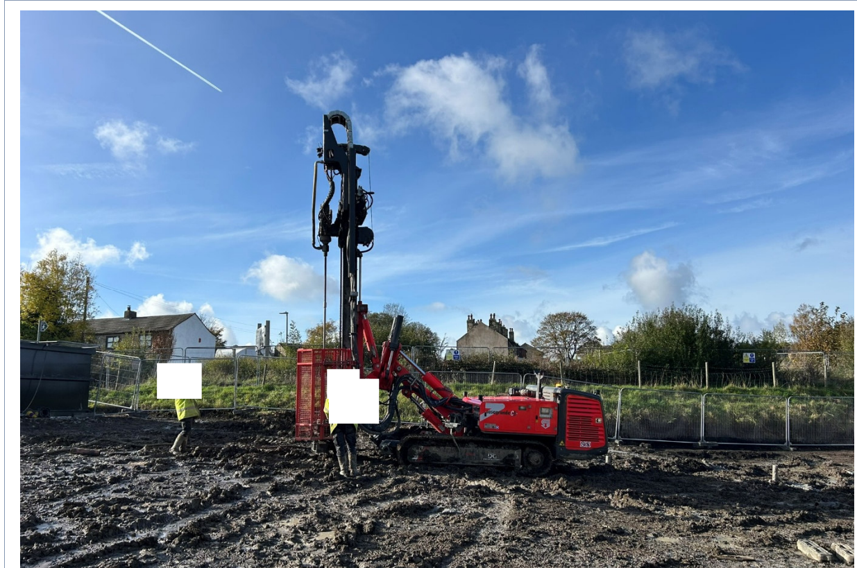
Photograph 4 – Drill and Grout works
