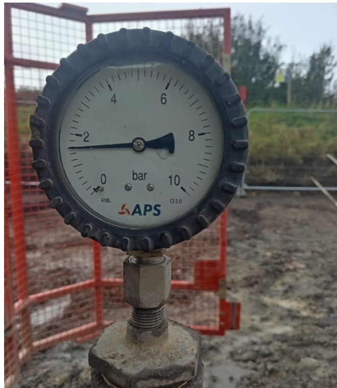
Photograph 8 – Pressure gauges during grouting of TH2.
