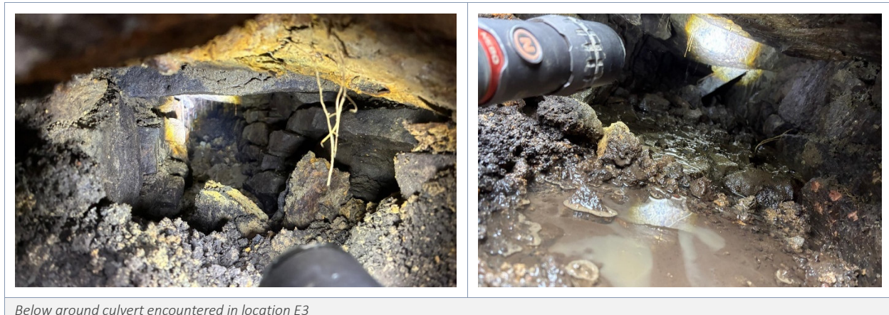
Below ground culvert encountered in location E3
