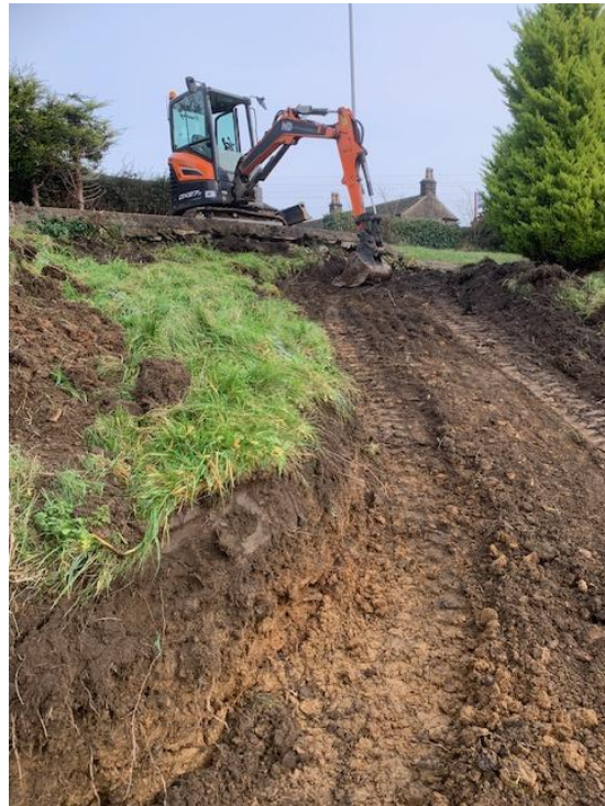
Excavating road for drilling rig access
