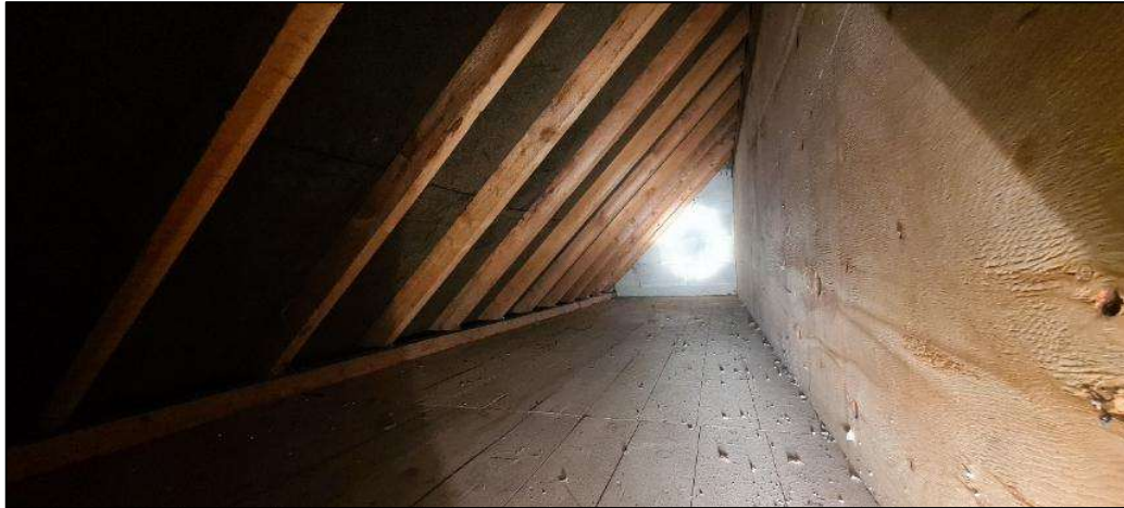
Plate 11. The storage space at the eaves of Building 2
