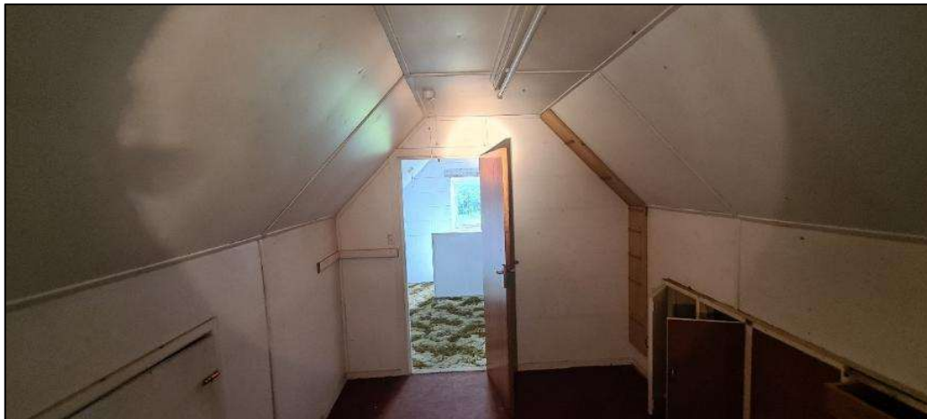
Plate 10. The interior of the first floor of Building 2.
