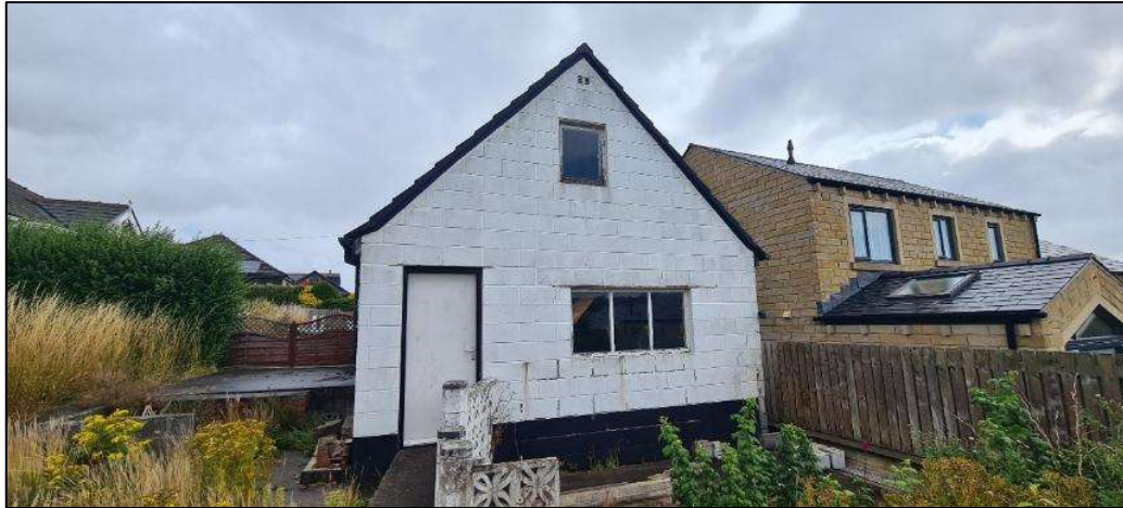
Plate 9. The southwest elevation of Building 2
