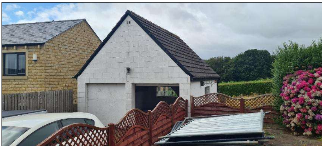
Plate 8. the northeast elevation of B2
