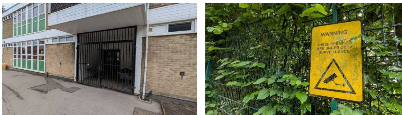
Figure 05 Gated recess to southwest elevation
