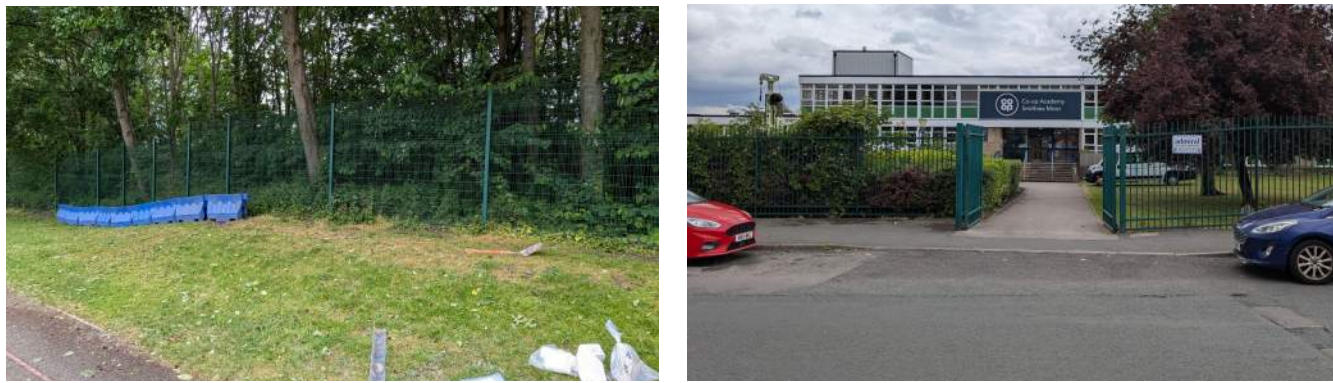
Figure 03 Weldmesh (left) and railing (right) outer site boundary treatments
