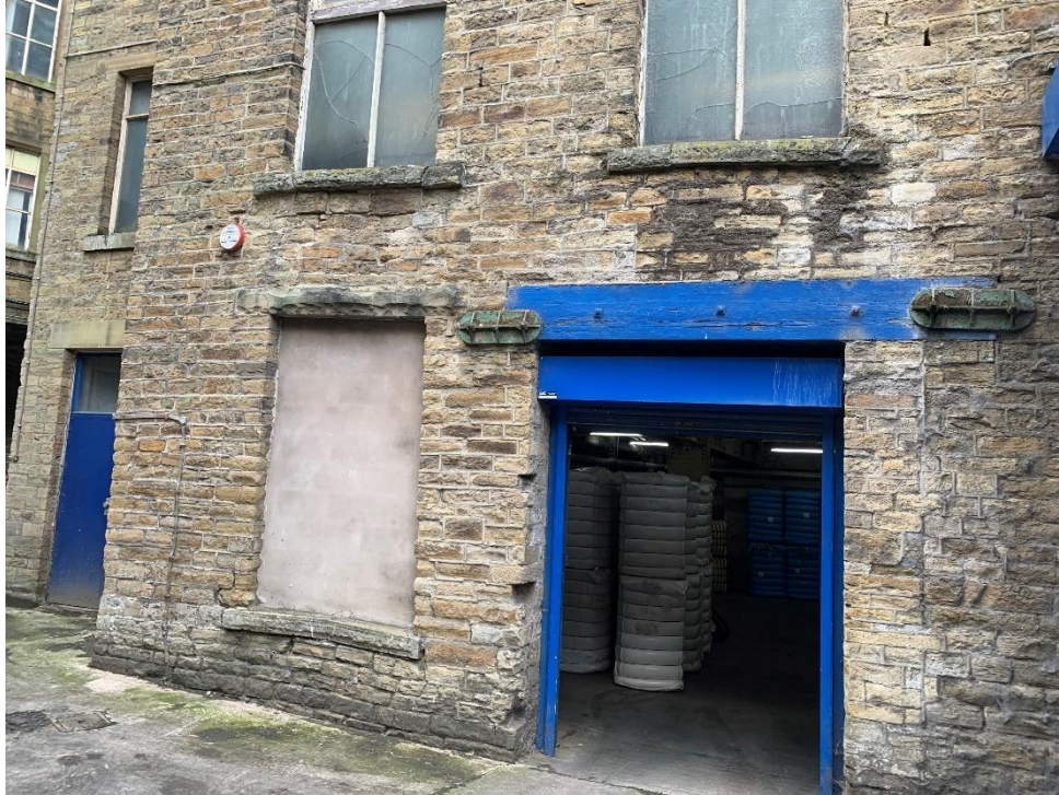
Figure 3 - Photograph of Existing North-East Facing Elevation, where new Doorset is to be built in place of existing window aperture
