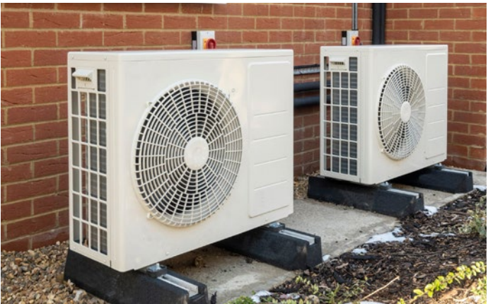
Typical air source heat pump unit
