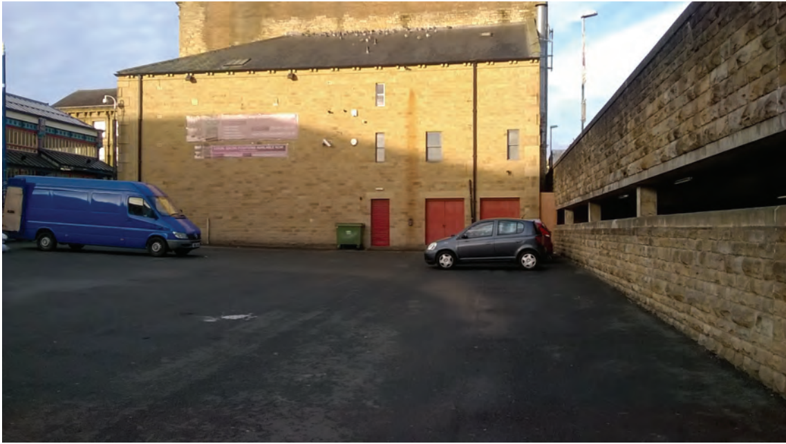
Photo 1 : Area of Development. Two storey car park on the right.
