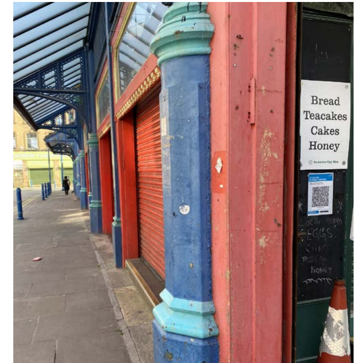
Photograph of existing opening details
