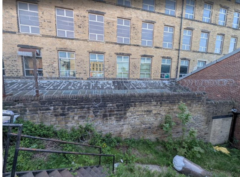
Photo 2. View of western wall of building.
