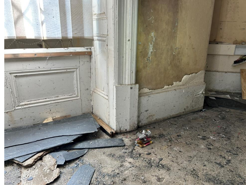
Photo 9.3: Close-up of window architrave & panelling alongside modern skirting boards
