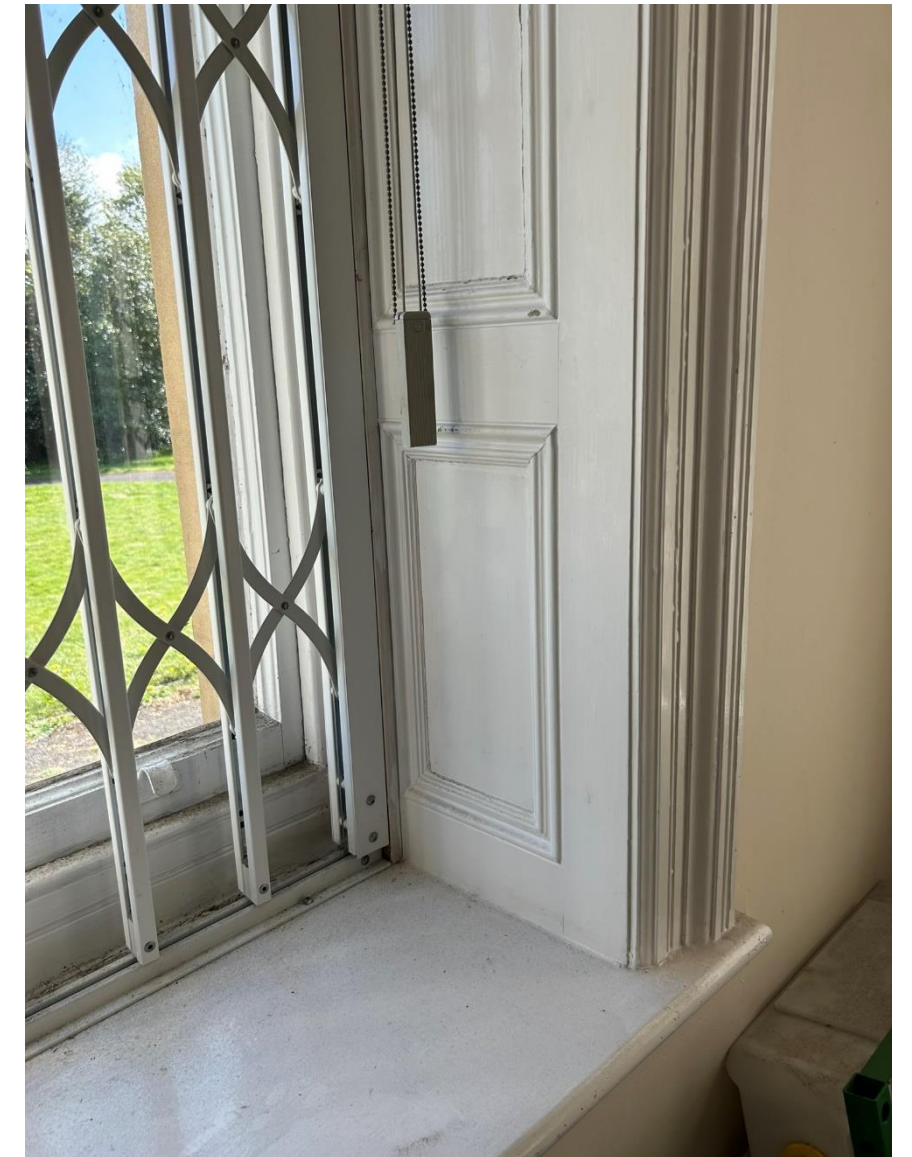
Photo 3.3: Historic architrave & panelling to window
