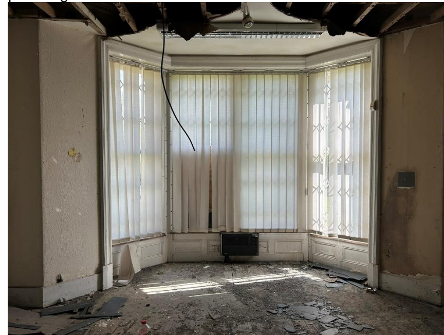
Photo 9.2: Cantered bay window including historic architrave & panelling
