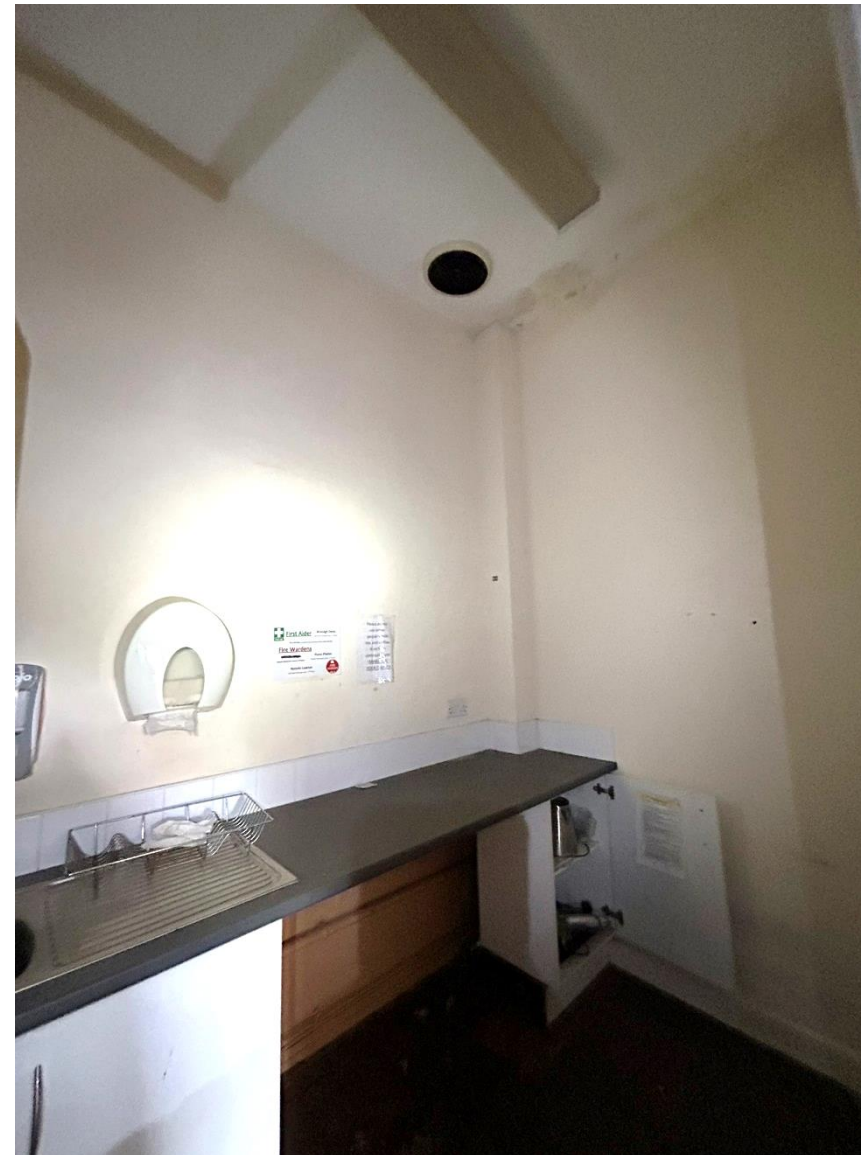
Photo 17.2: General view (wide angle)
