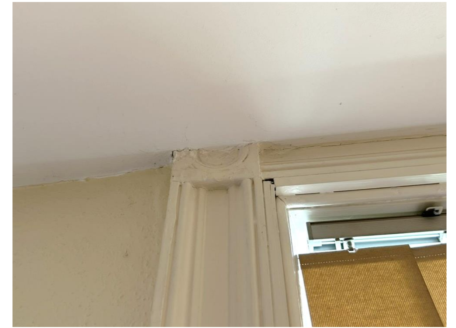
Photo 5.3: Older architrave detail to former front door (now window)
