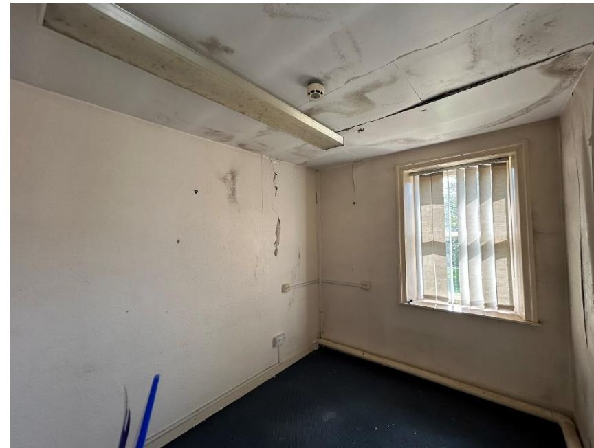
Photo 13.2: General view (wide angle)
