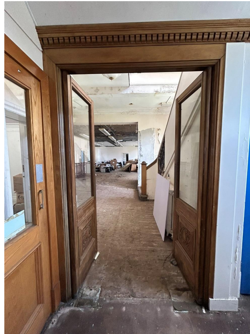
Photo 1.2: Double doors – probably historic but not in original location. Door to left modern
