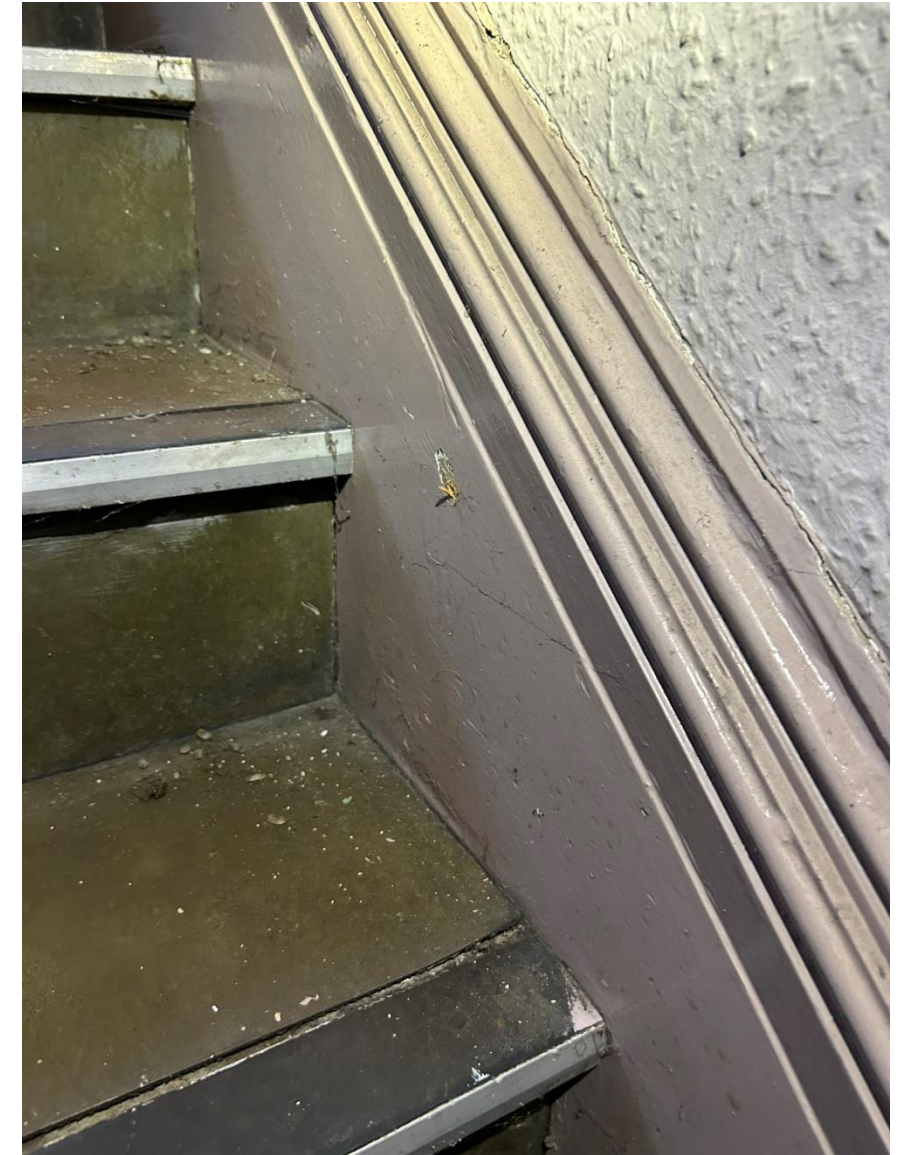
Photo S: Historic stringer along with vinyl clad treads & risers
