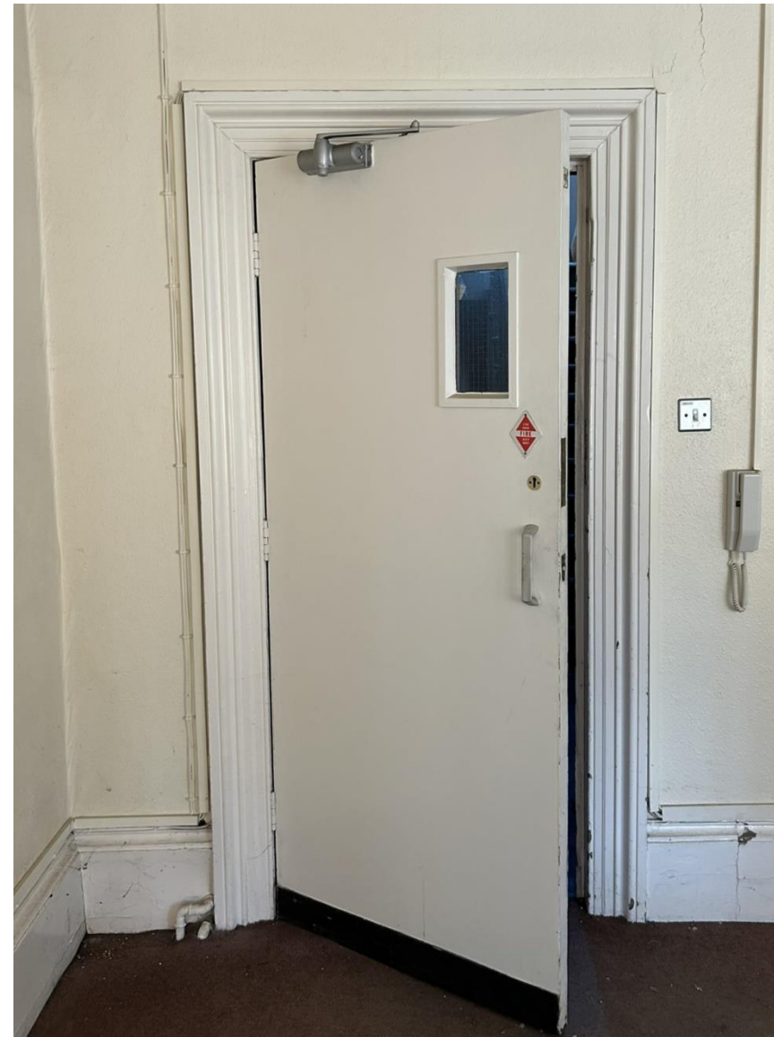
Photo 5.2: Door to rear hall along with historic architrave & skirting board
