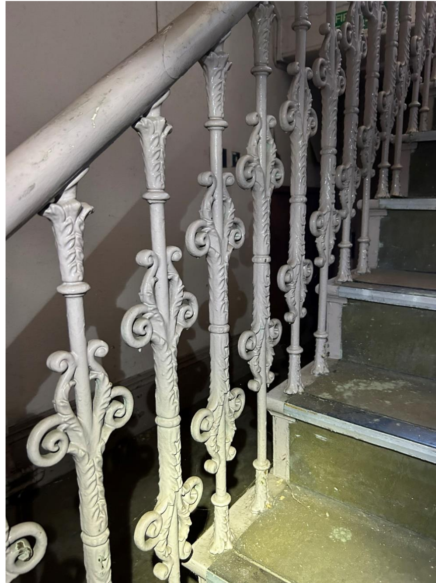
Photo: R: Cast iron spindles & wooden handrail
