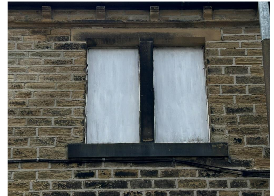
Photo F: Typical window detail to outbuilding, including simple chamfered lintel
