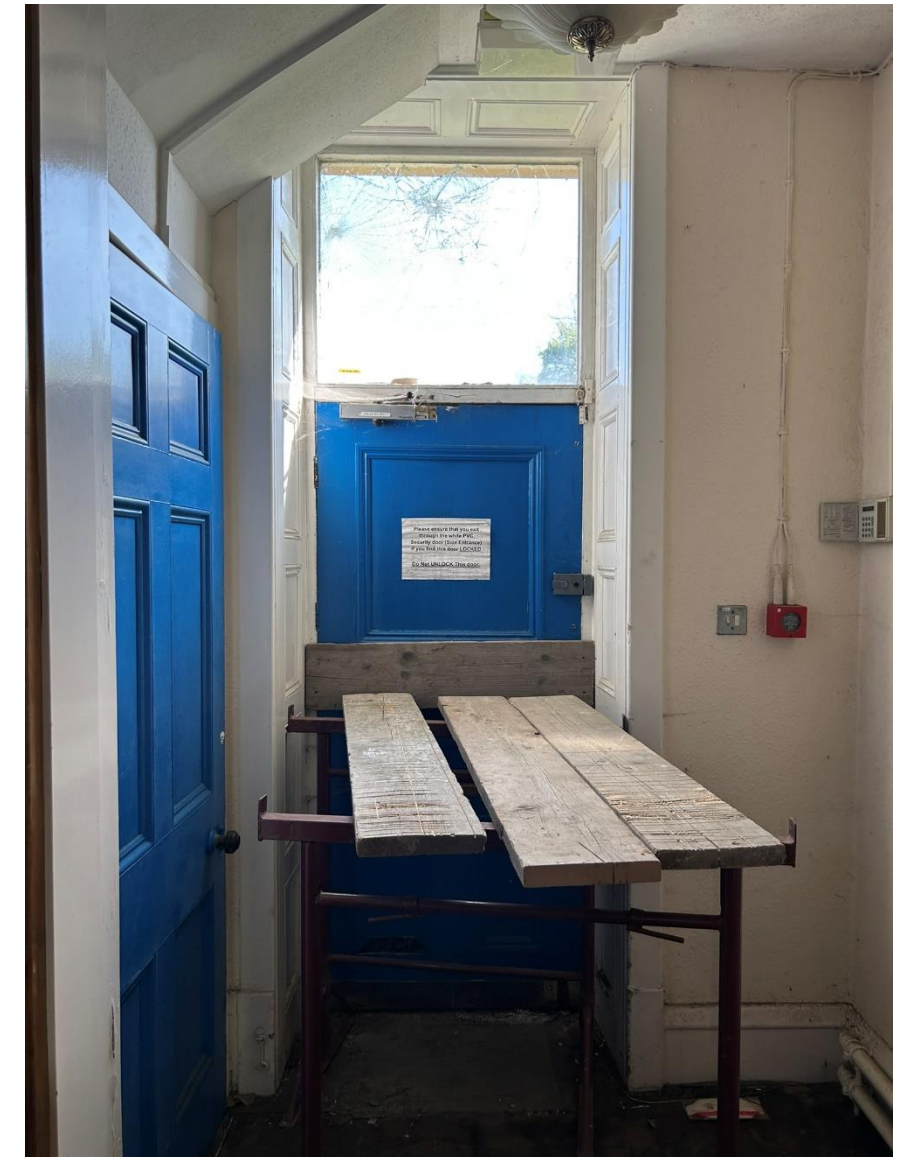
Photo 1.3: Entrance door, panelling & 6 panel door to cupboard under stairs
