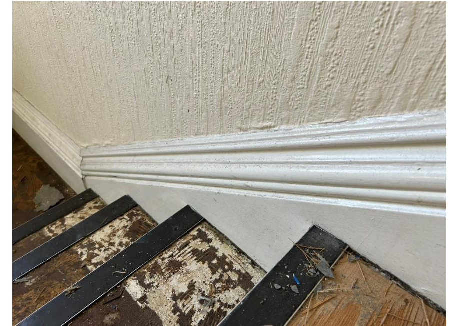
Photo P: Historic stringer & skirting board to intermediate landings
