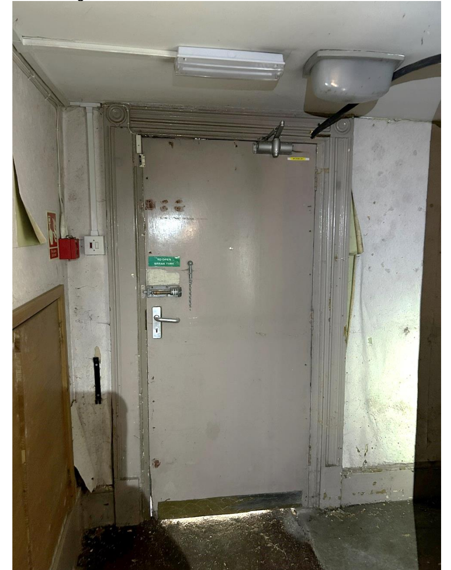
Photo 6.3: External door along with historic architrave & modern/low skirting boards
