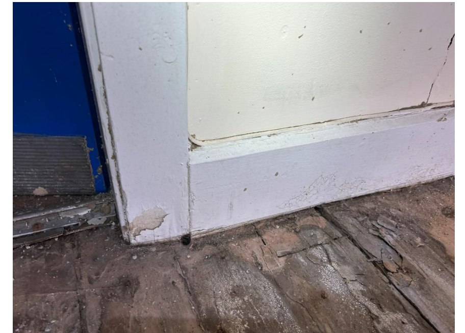
Photo 19.3: Close-up of modern architrave & skirting boards
