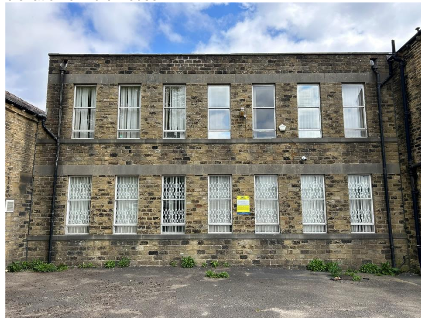
Photo D: Rear elevation of link extension that provides a good well matched supply of random coursed stone to make good the north elevation of Acre House
