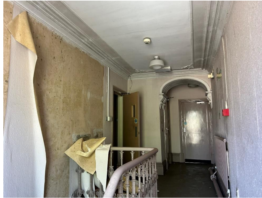
Photo 14.2: General view (wide angle)
