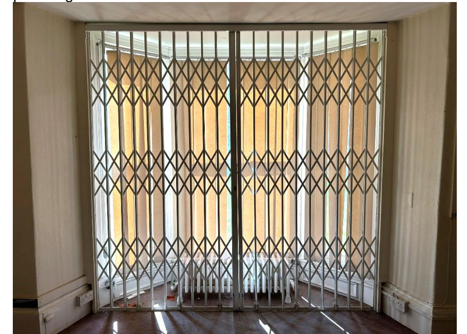
Photo 5.4: Cantered bay window including historic architraves and panelling under
