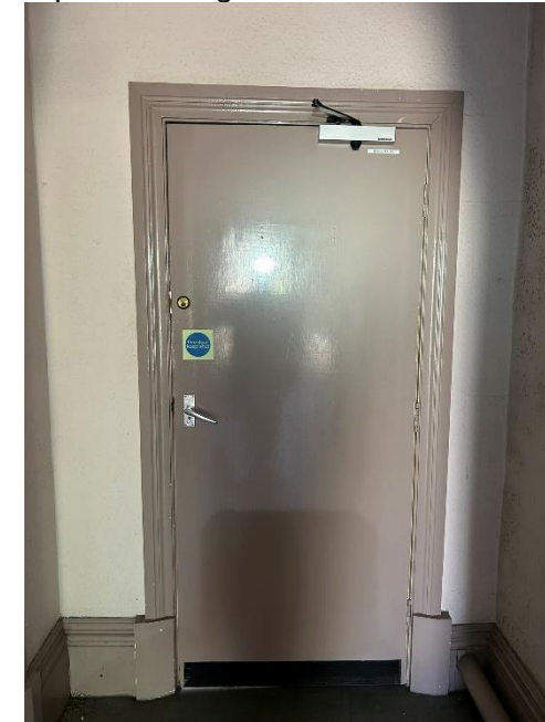
Photo 14.4: Modern door & modern architraves but with historic or replica skirting boards
