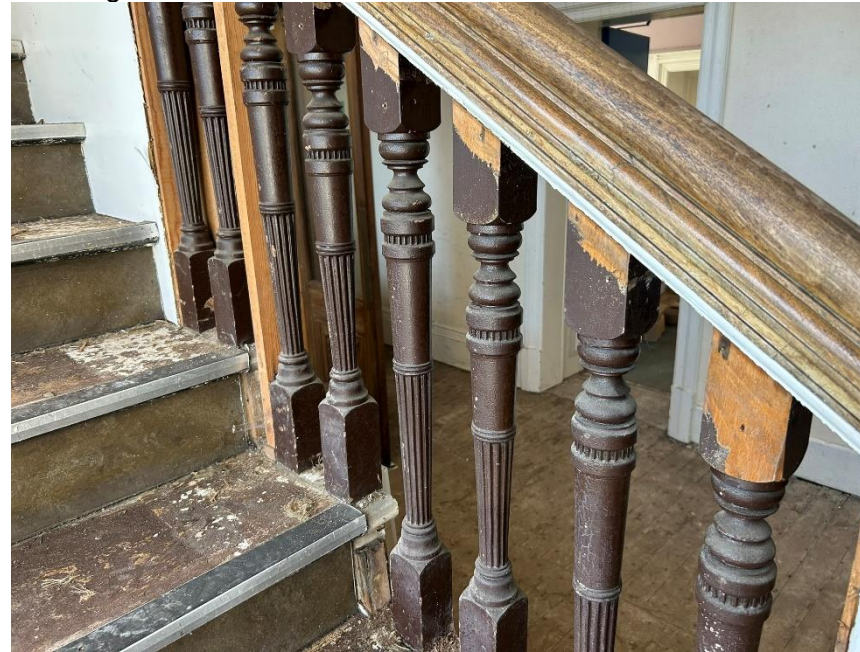
Photo N: Hardwood handrail & painted spindles with modern cladding removed
