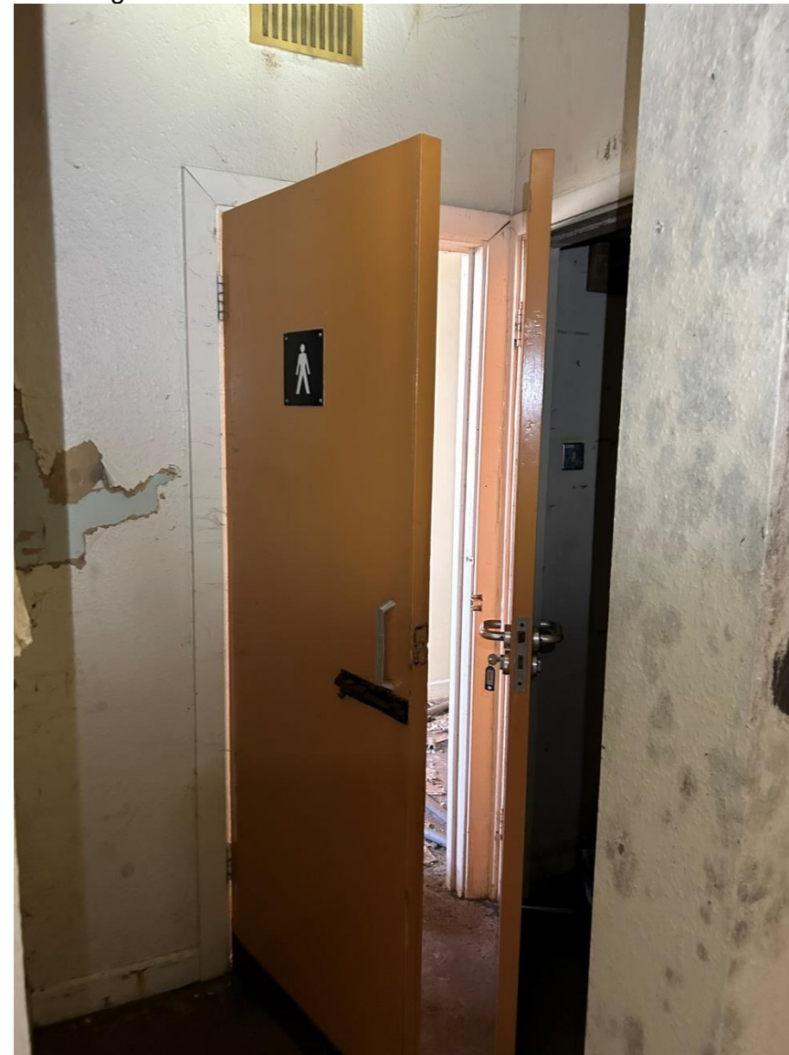
Photo 8.2: Door to toilet & cupboard along with modern architrave & skirting boards
