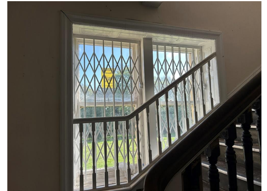
Photo 2.3: Stair window with historic architrave & panelling
