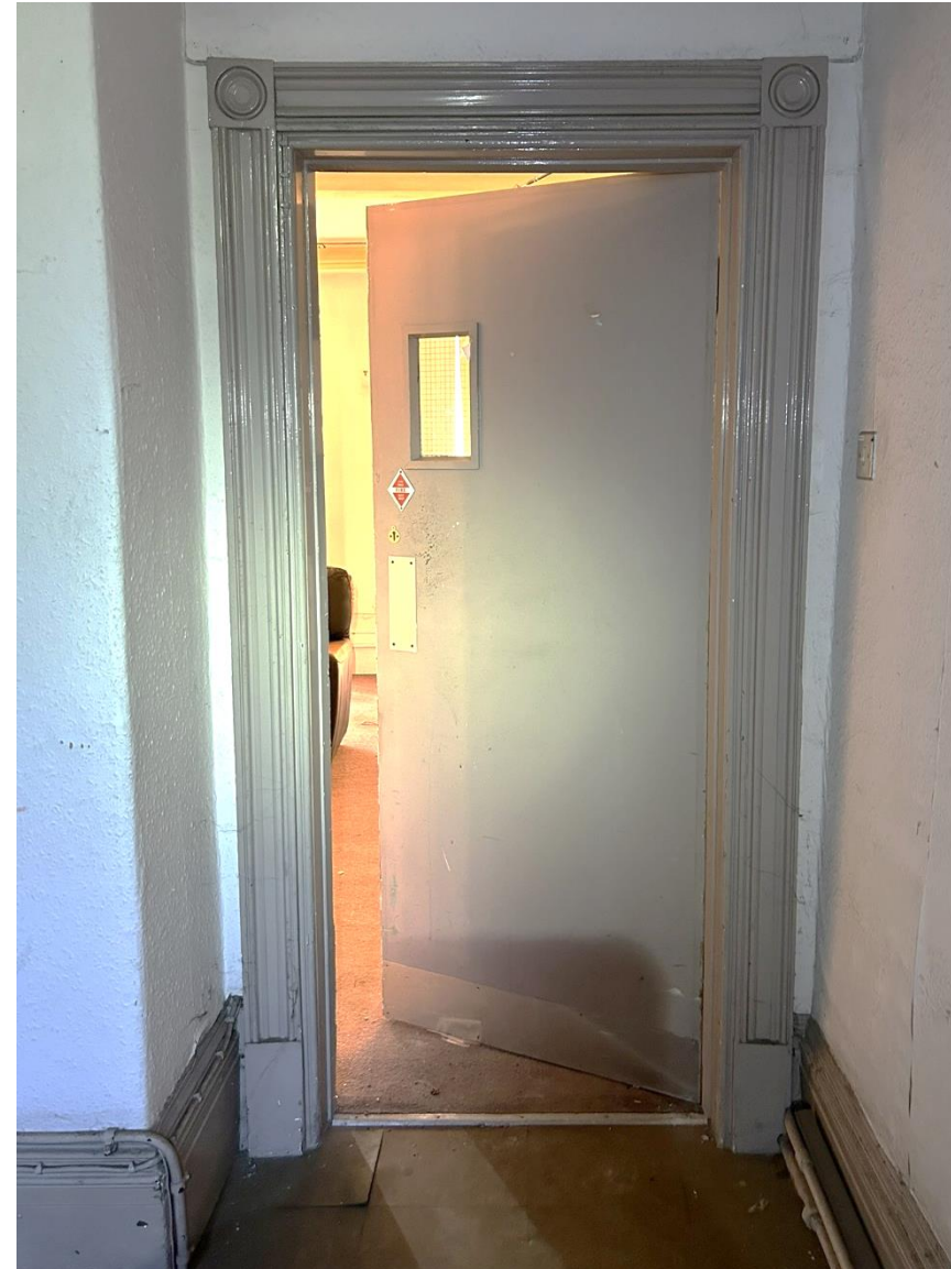
Photo 6.2: Door to scullery along with historic architrave & skirting board
