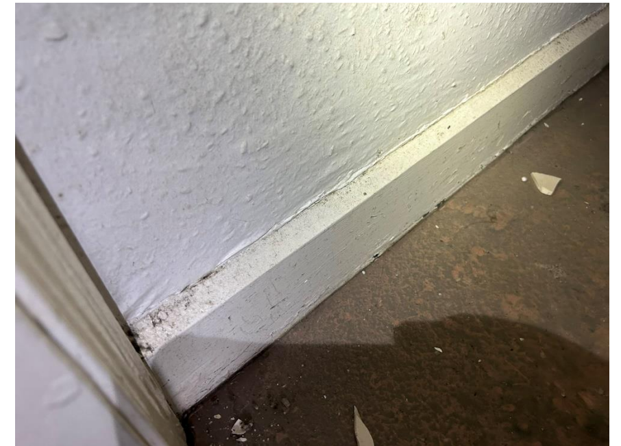
Photo 18.3: Modern skirting boards (where existing)
