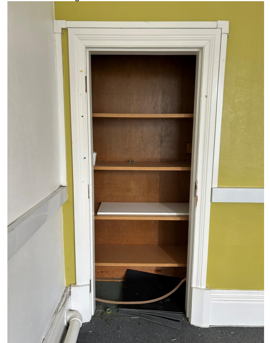
Photo 12.3: Former door to passage along with modern architraves but historic skirting boards
