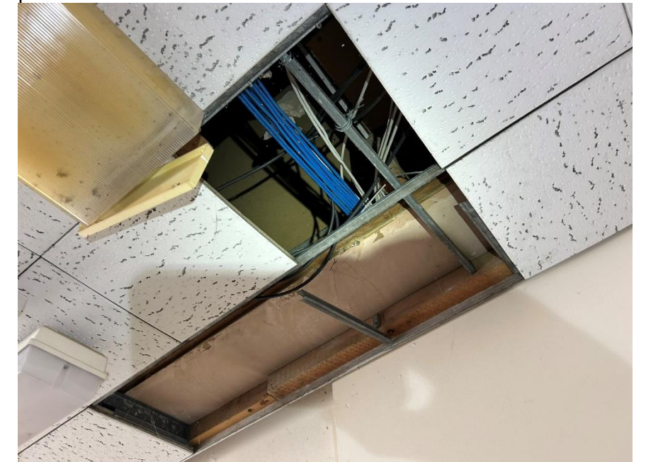
Photo 19.4: Removed ceiling tiles reveal no historic cornice or other plasterwork
