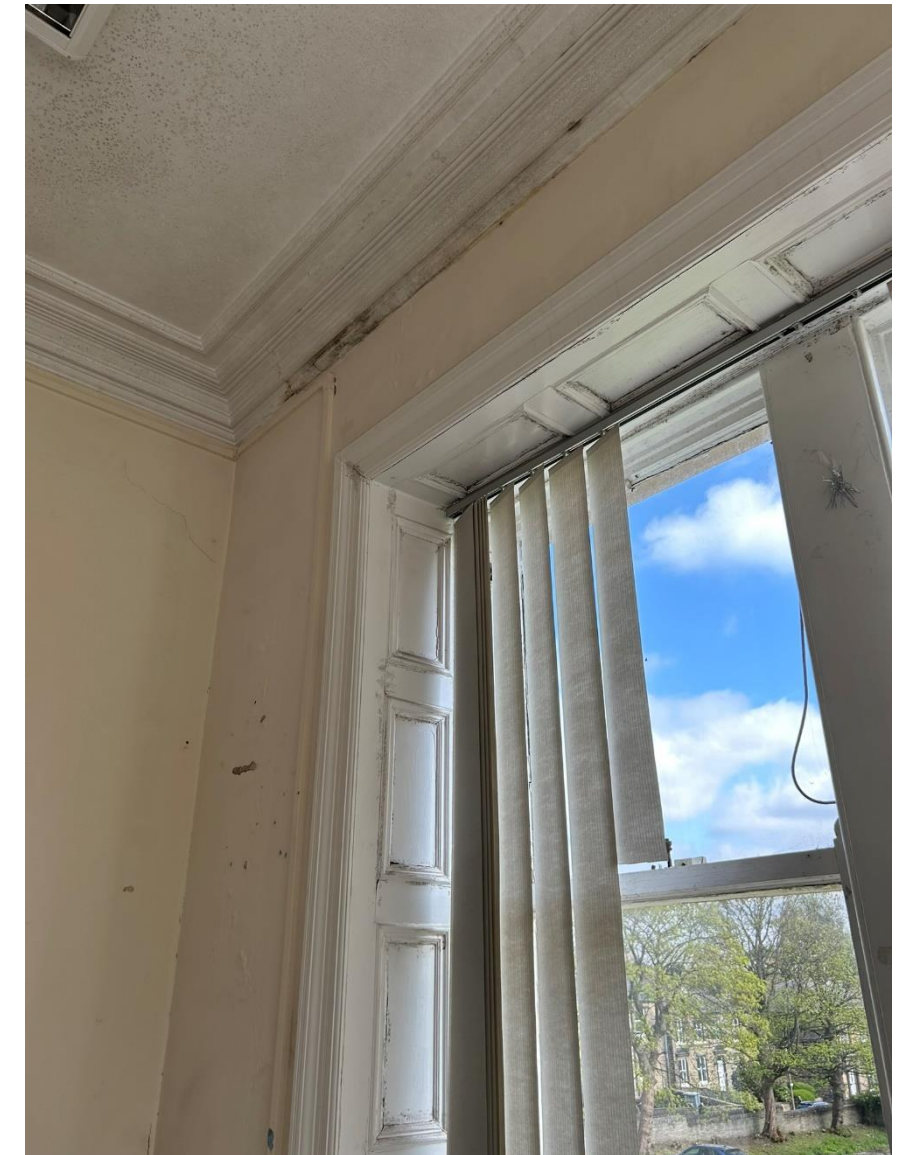
Photo 11.3: Close-up of window architrave & panelling alongside cornice
