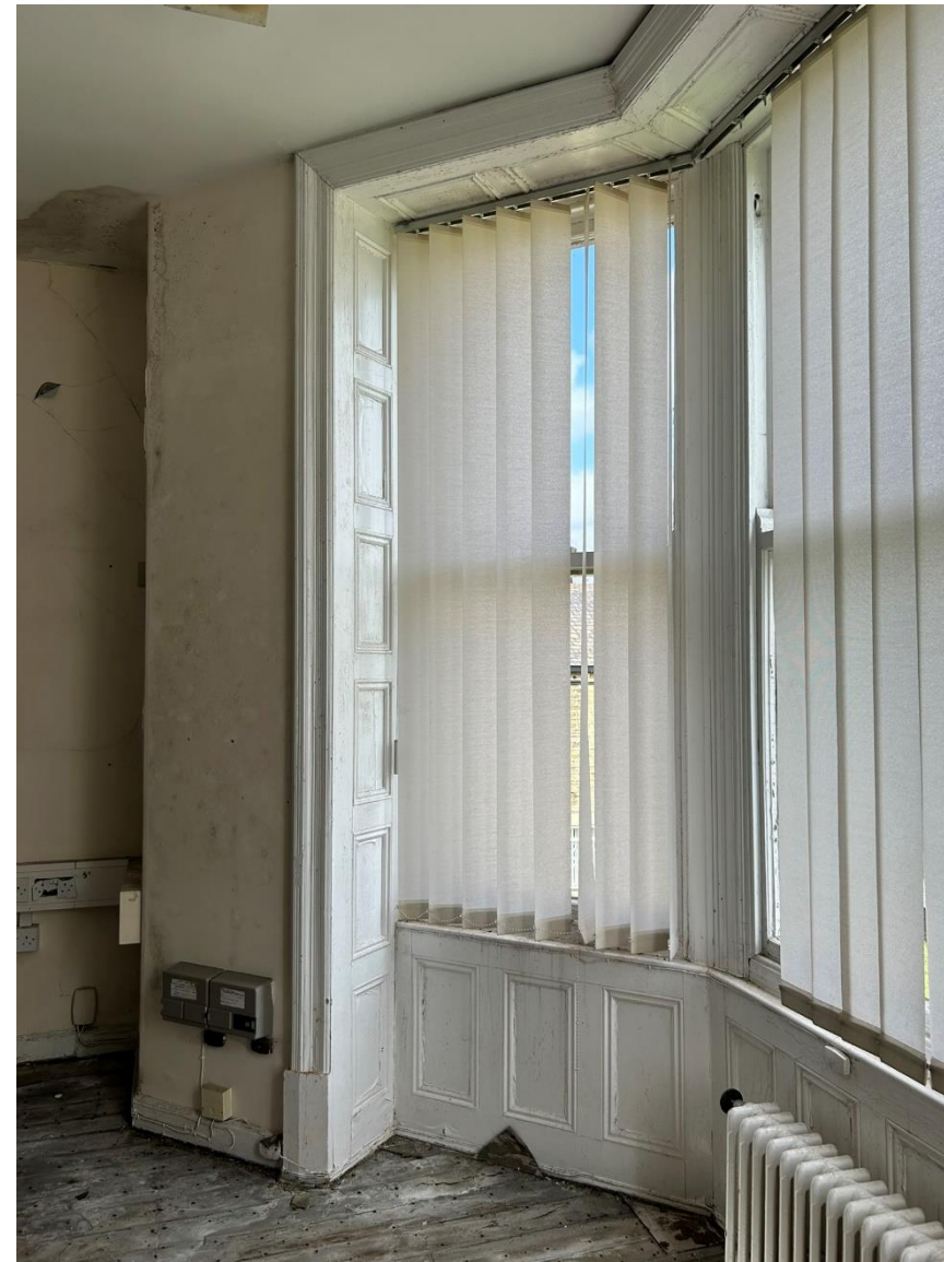
Photo 19.2: Close-up of panelling to cantered bay window
