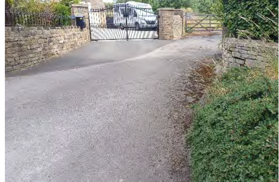
Photograph 4: Driveway present in the southwest of the Site (04.07.2025)
