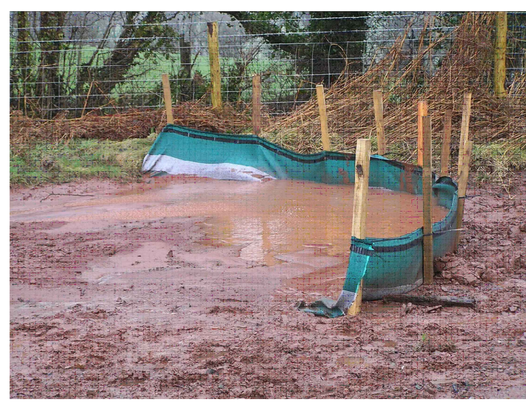
HY-TEX TERRASTOP SILT FENCING TO BE INSTALLED TO MANUFACTURERS SPECIFICATION (Refer to manufacturers installation guidance)
