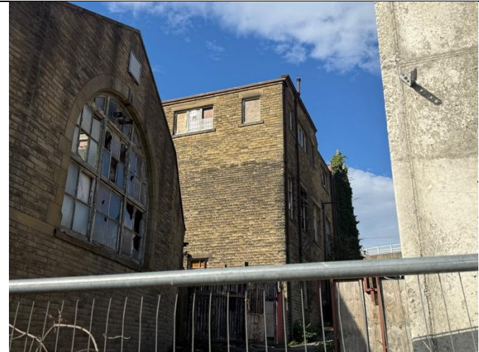
Southern elevation of B1
