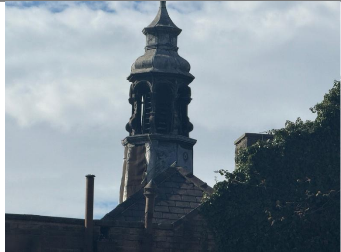
Full view of tower structure on B1
