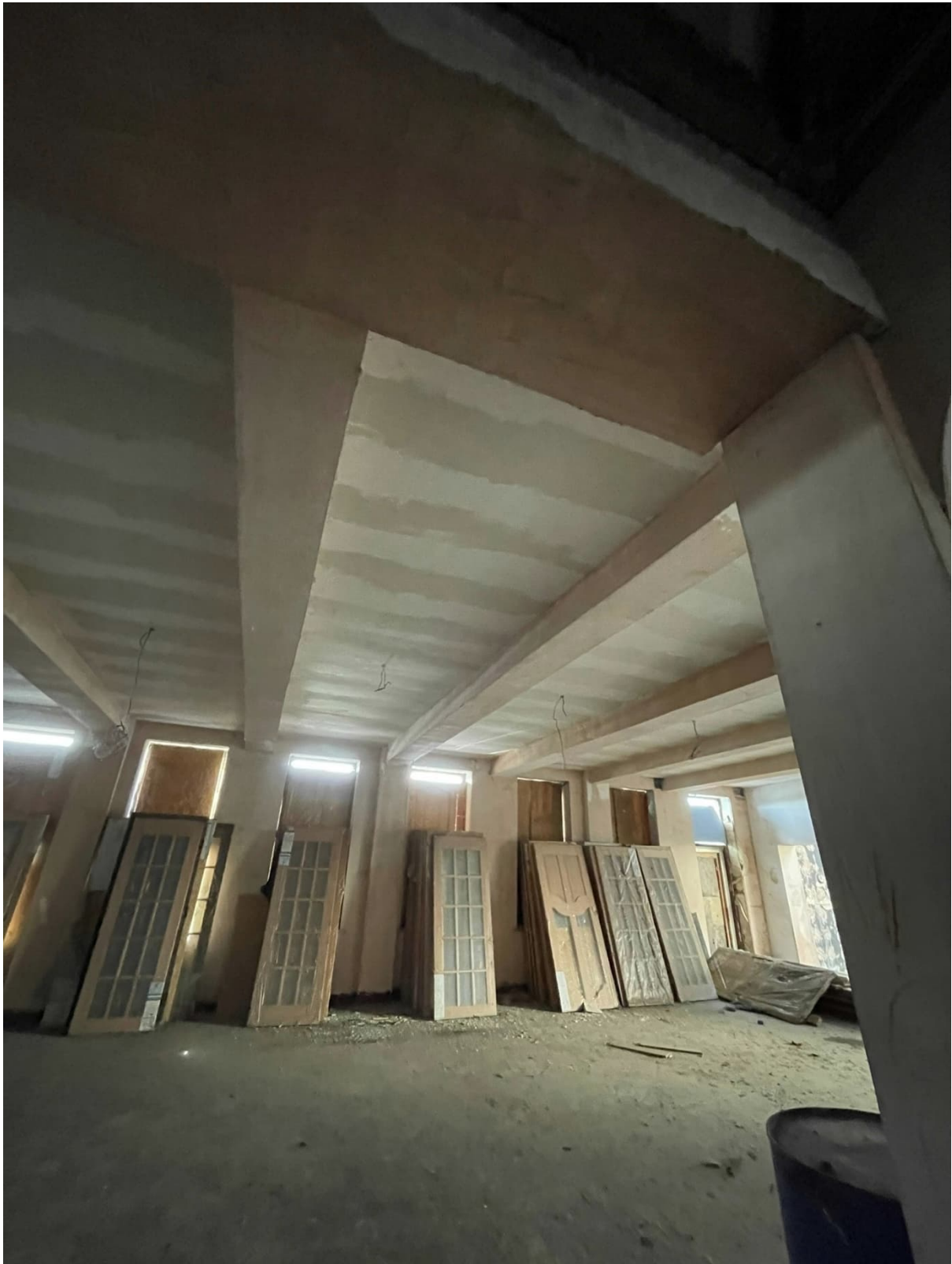
Close centre downstand beams under first floor hall.
