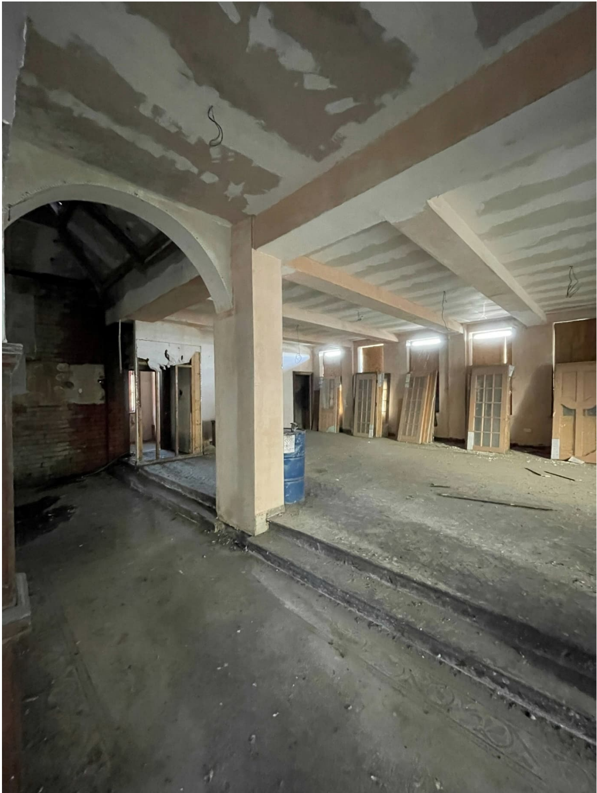
Downstand beams, likely from previous internal alterations.
