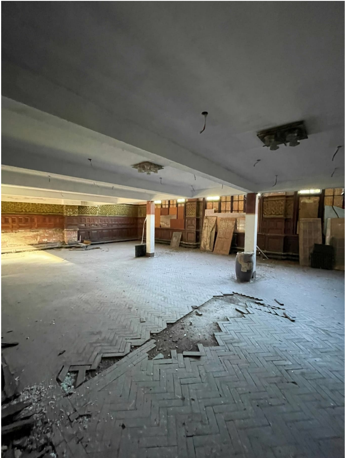
Mezzanine floor with downstand beams and columns.
