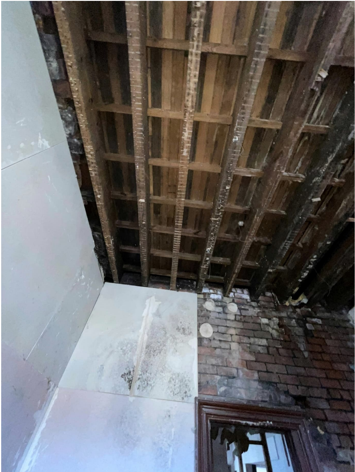
First floor joists over toilets.
