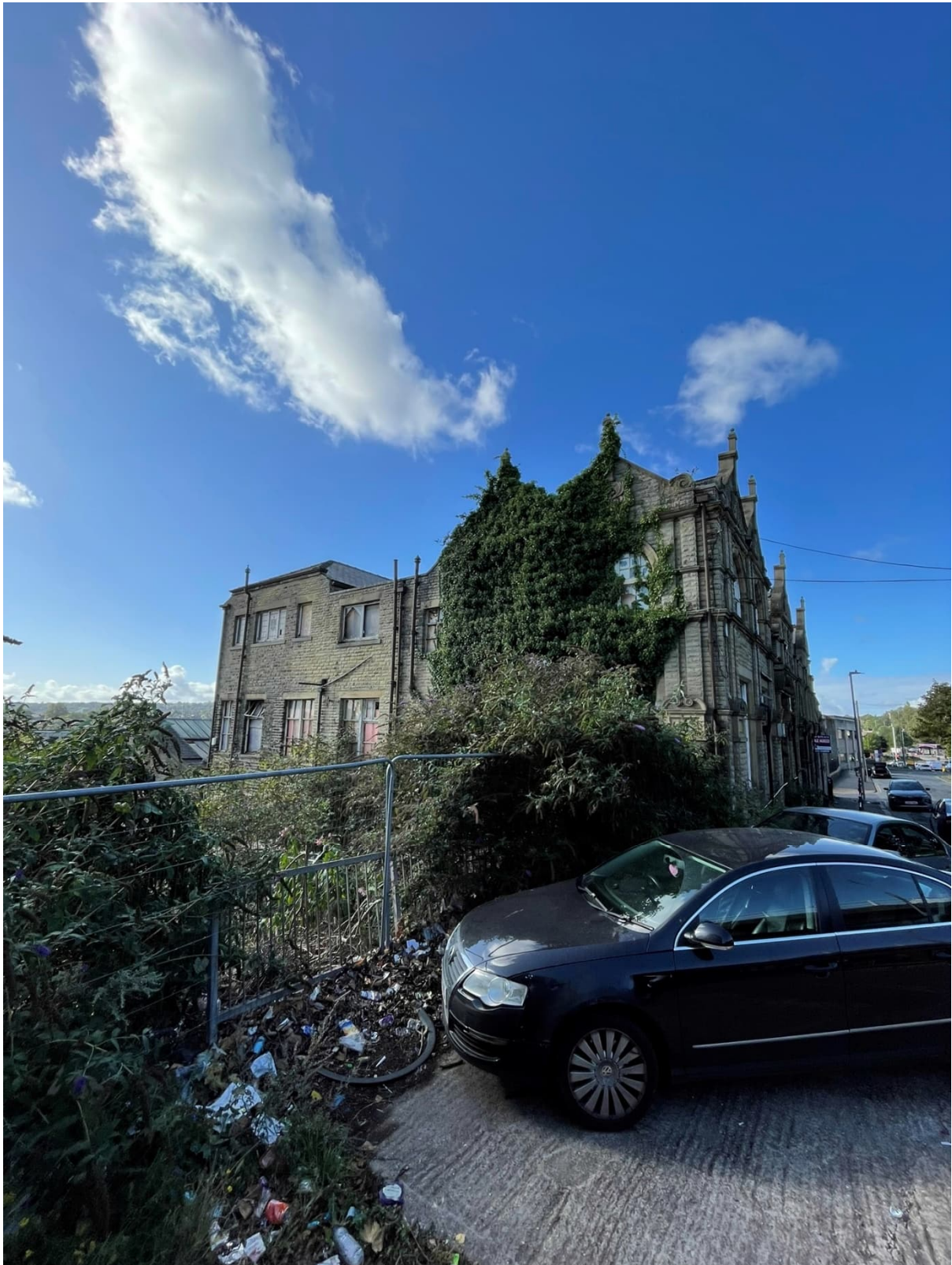
North East elevation, climbing vegetation.
