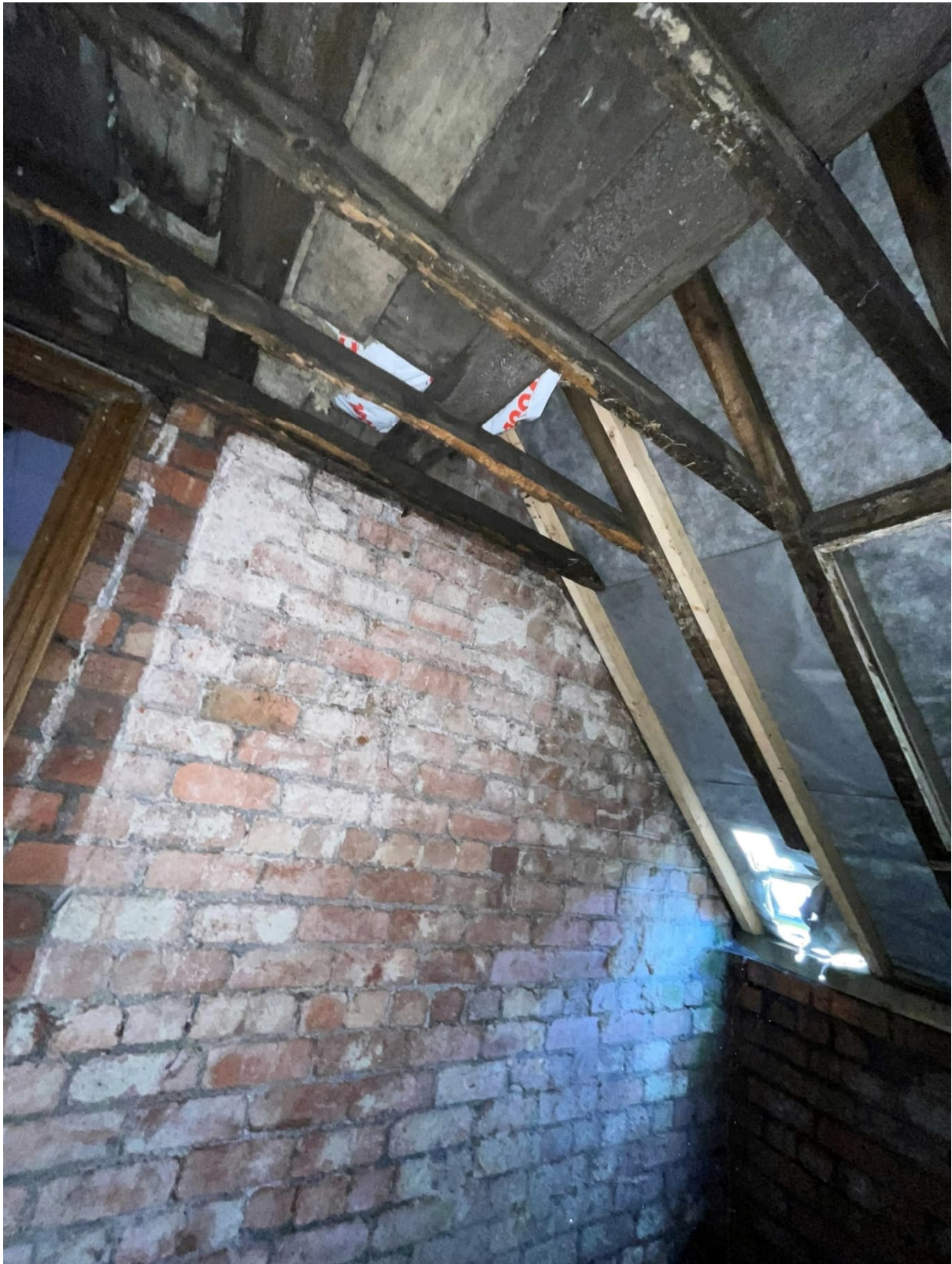
Purlin supporting rafters, sitting on wall to be removed.
