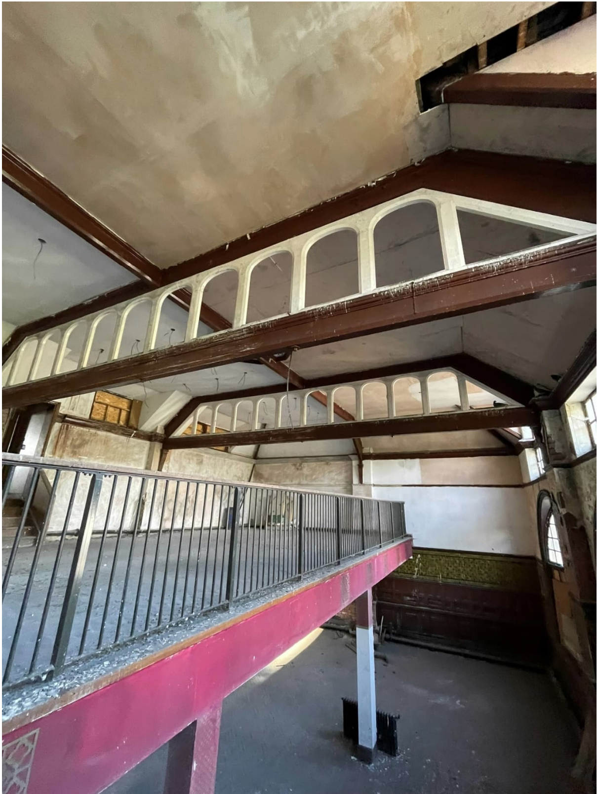
Trusses over first floor mezzanine in hipped roof.
