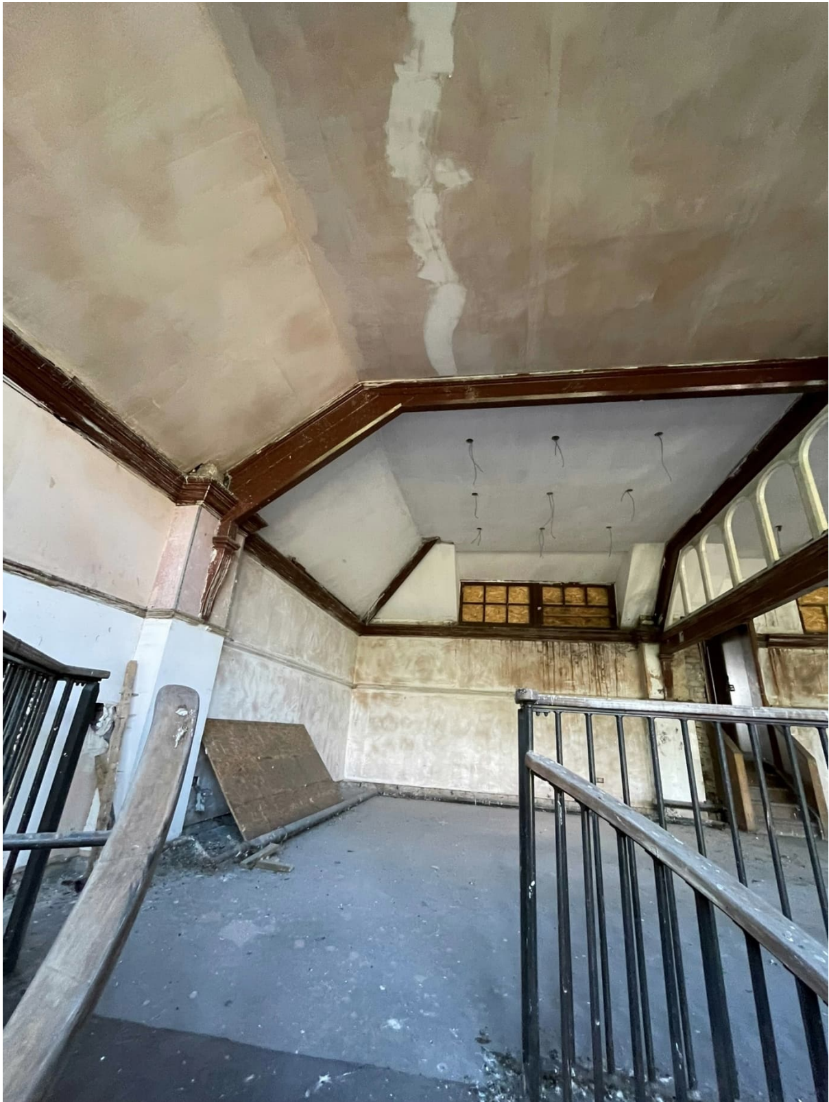
Masonry piers for truss bearing.
