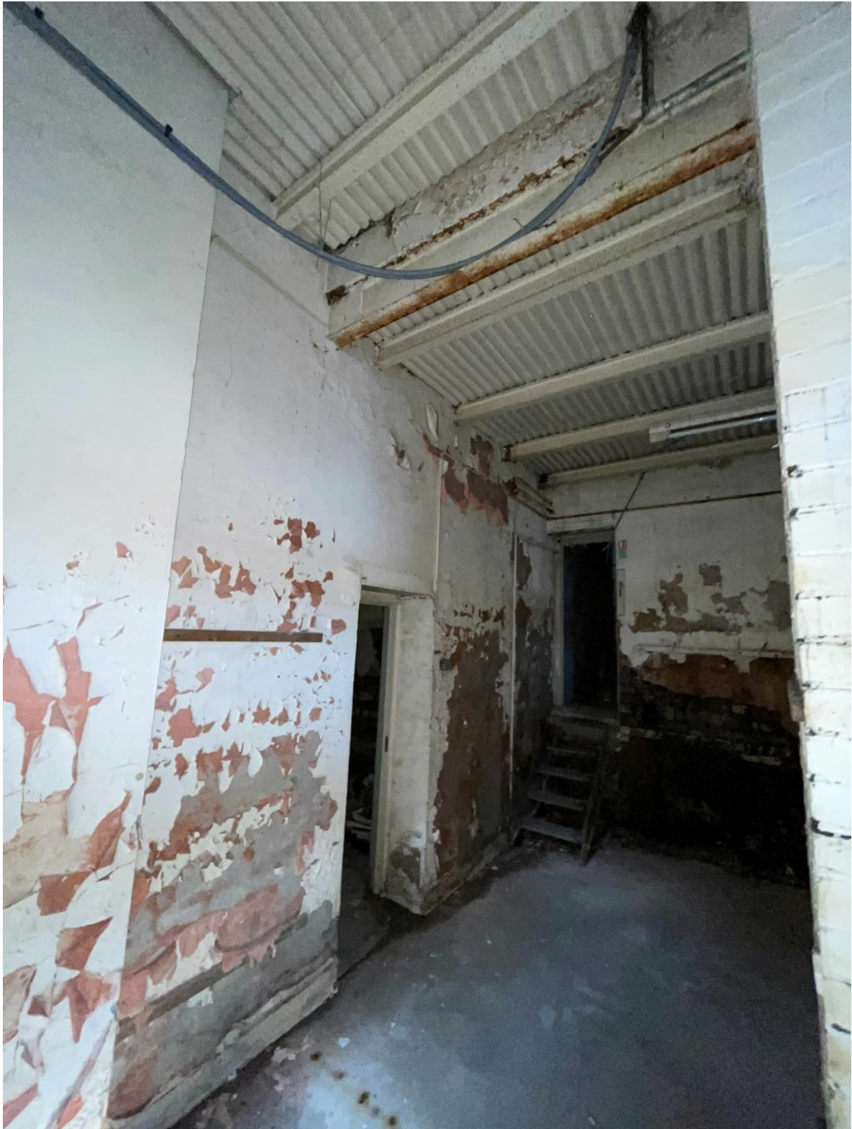
Steelwork gillage and sheeting to underside of suspended ground floor.
