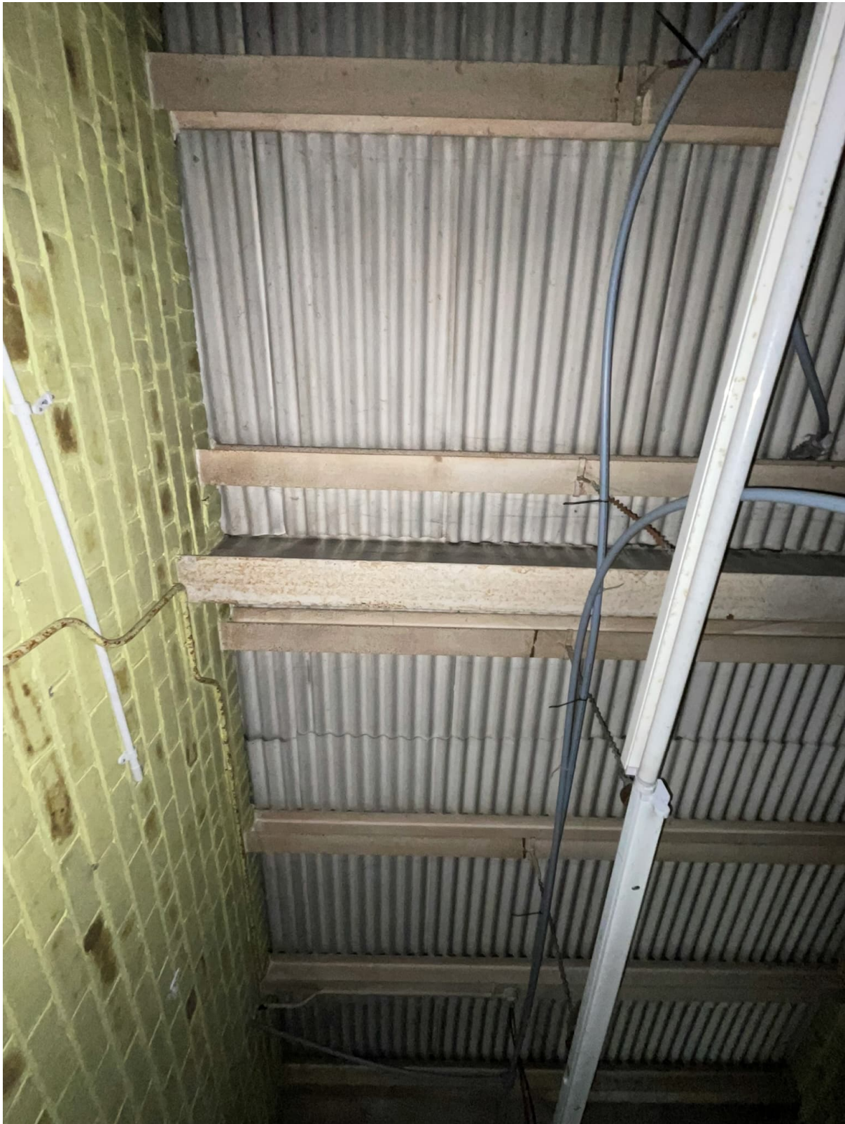
Steelwork grillage & sheeting to underside of ground floor.
