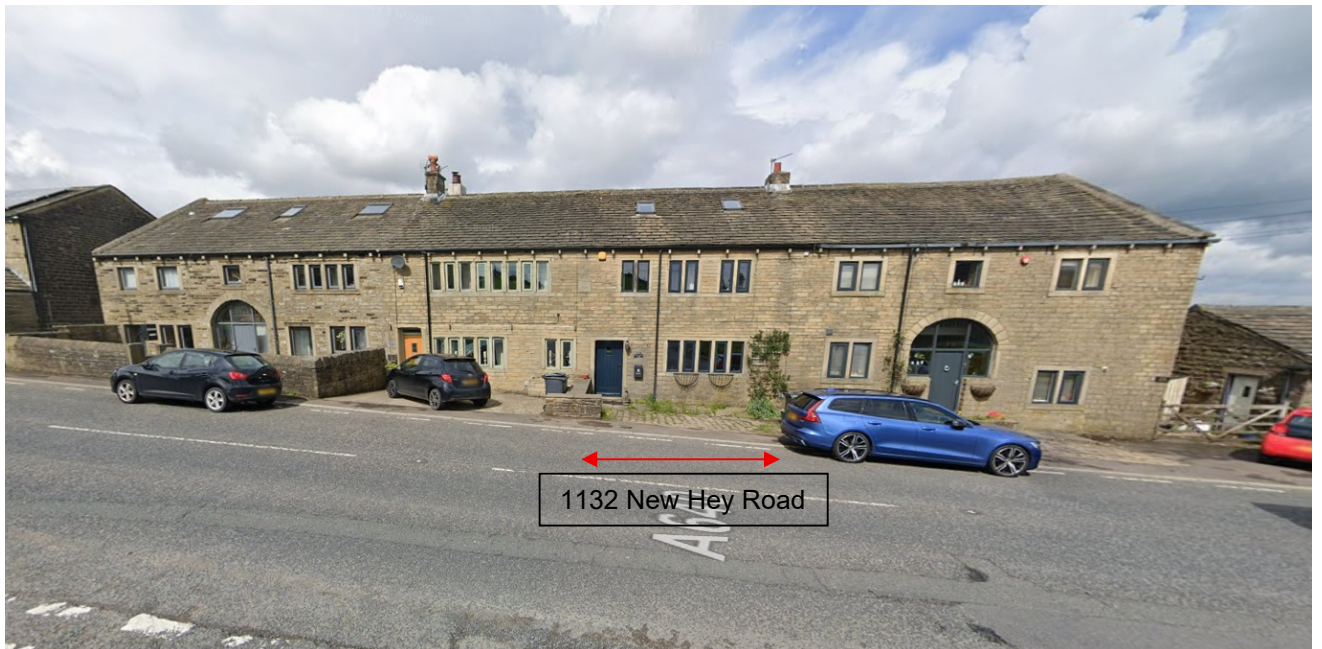
Front elevation of 1130 (Hardenby Farm) to 1136 New Hey Road
