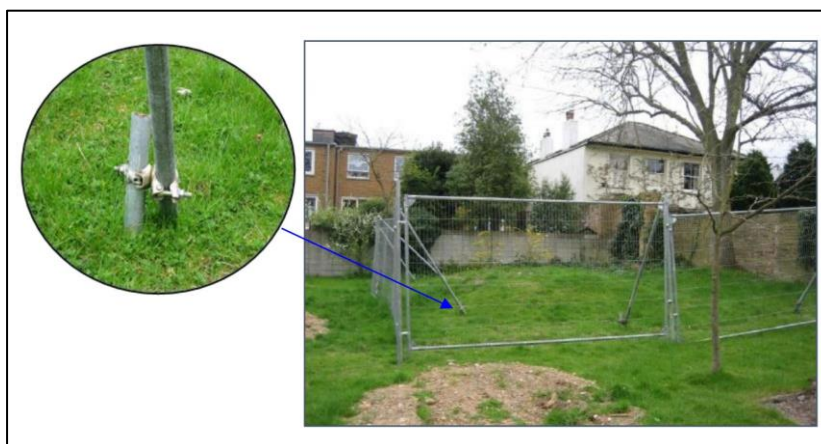
Figure 2.1: Example of mesh welded type barriers in-situ.
