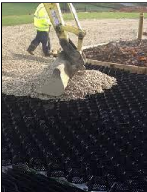
Figure 2.4: Cellweb ® geo-cellular confinement sheets being infilled with 4/20 mm clean, angular stone.
