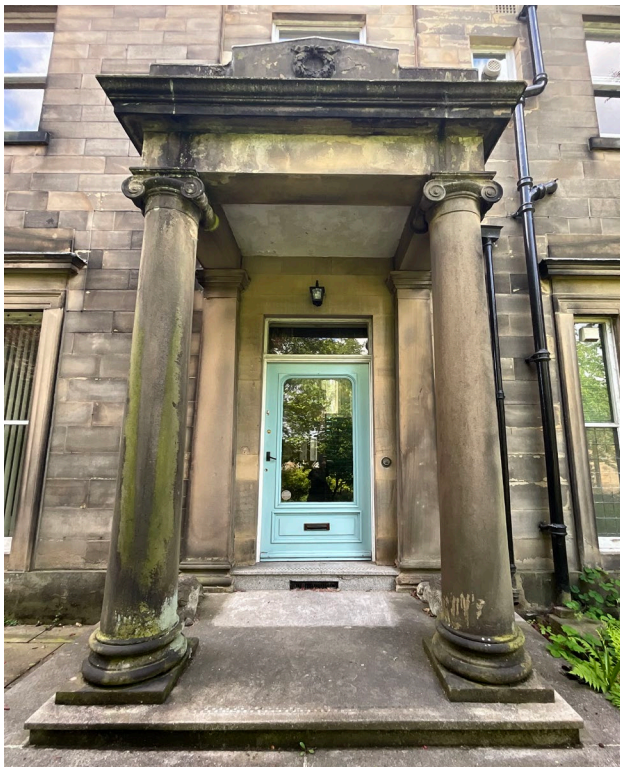
Figure 5: Grade II Listed Entrance Columns. View of the classical stone entrance portico, including the original columns which are Grade II listed. These features will remain entirely unaffected by the proposed change of use.
