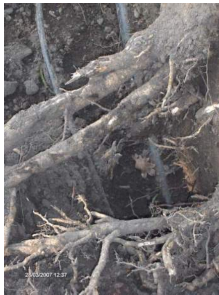
Typical root damage caused by excavation works
