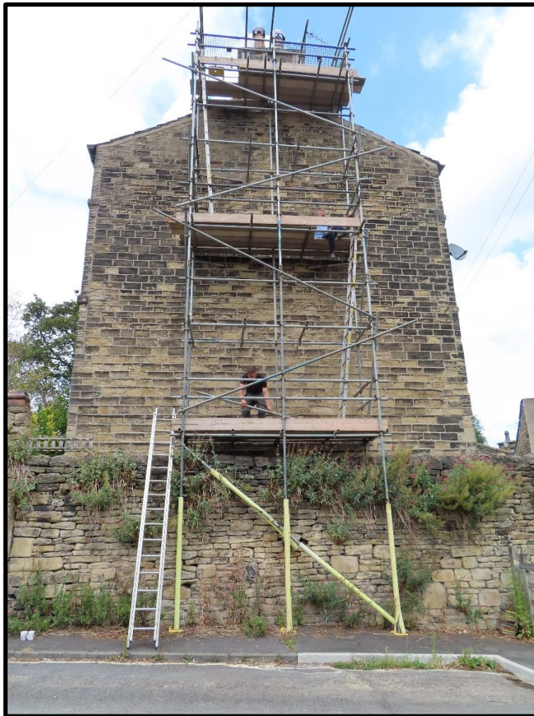
“ Elevation on gable with scaffold adjacent Westcroft Road”
