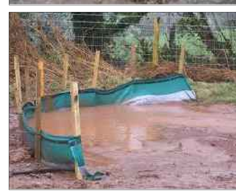
TYPICAL SECTION THROUGH HY-TEX TERRASTOP PREMIUM SILT FENCE (1:NTS)
