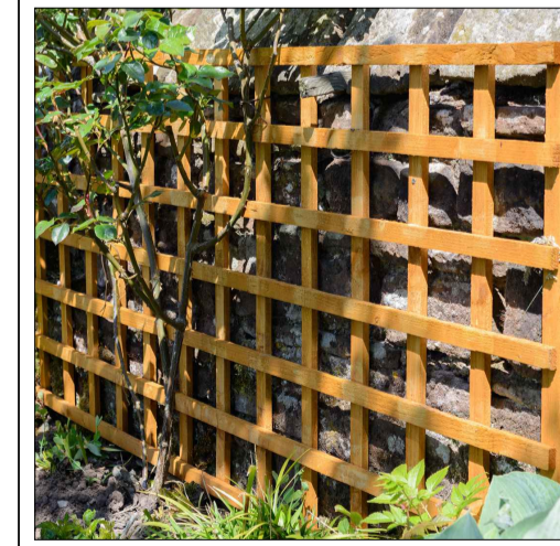
TIMBER 'CRIB'/TRELLIS FASCIA TO RETAINING WALL
