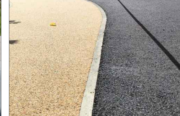
FLUSH CONCRETE EDGING
