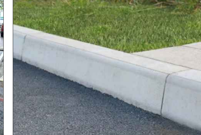
HALF-BATTER CONCRETE KERB
