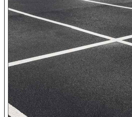
ASPHALT SURFACING WITH PARKING BAY DEMARCATION
