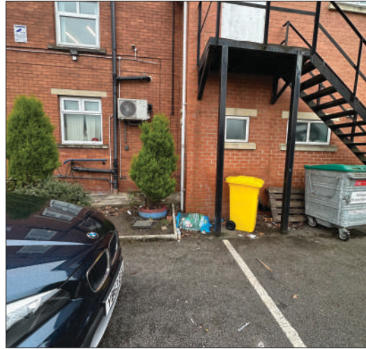
Existing side entrance into the rear building.
