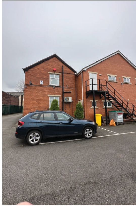
View to the rear within the parking area.
